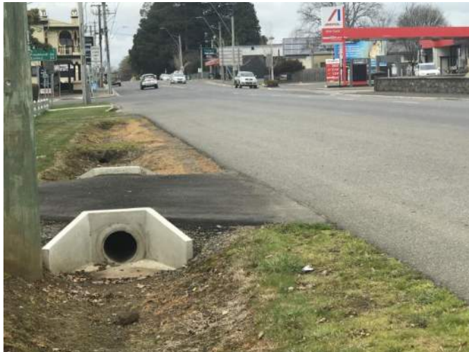
Figure 9 – Looking left along MVR from existing access
