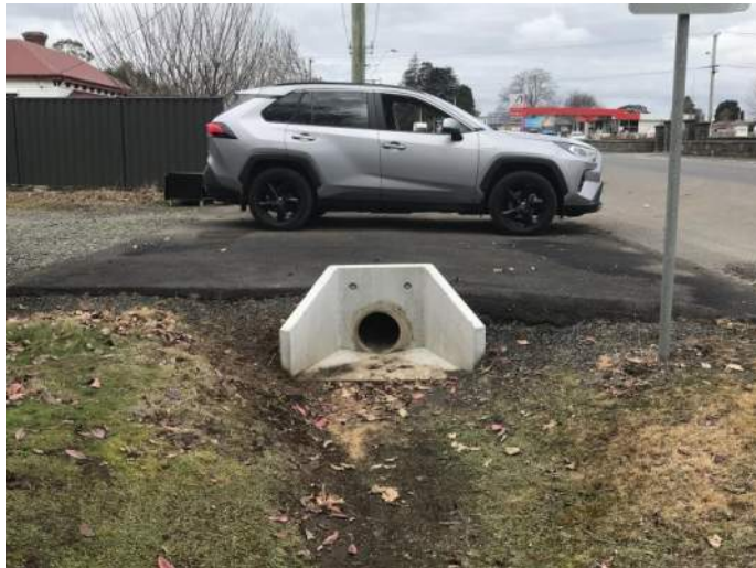
Figure 14 – Side elevation of 111a MVR driveway
