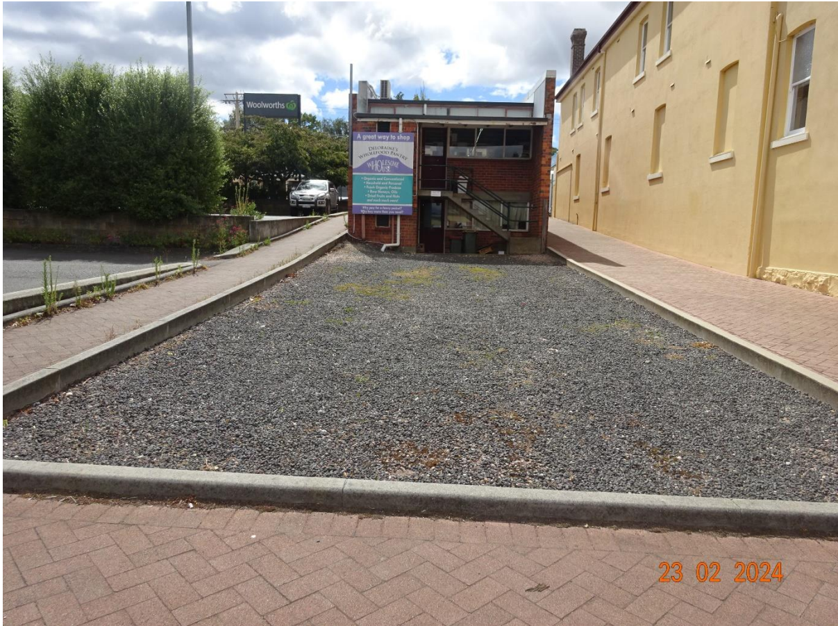
Figure 4: View of rear of 66 Emu Bay Road.
