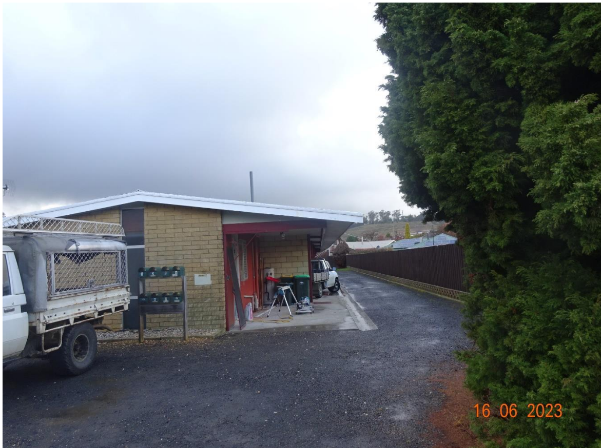
Figure 6: Photo of parking area for Unit 1 and shared driveway to the right.
