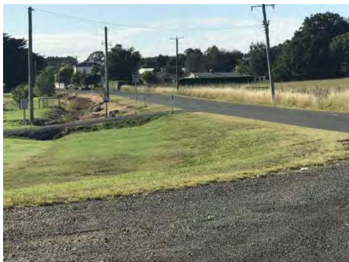
Figure 18 – Looking left along Meander Valley Road from Porters Bridge Road
