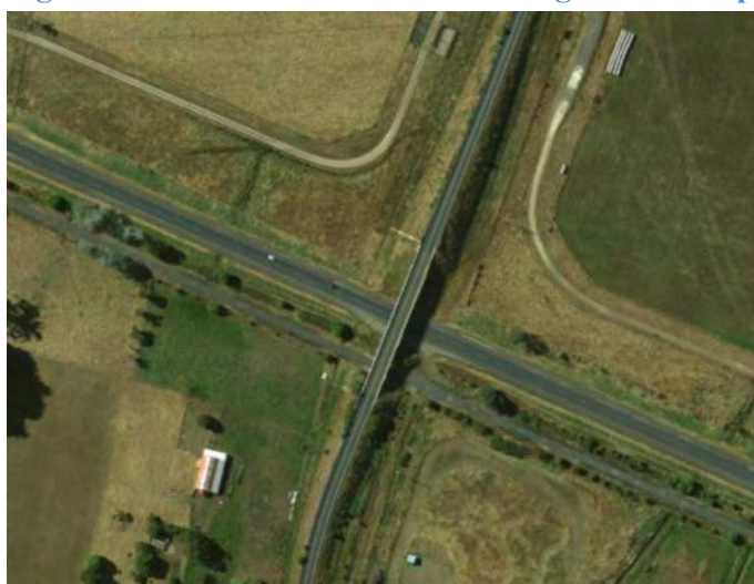
Figure 22 –Aerial view of Porters Bridge Road overpass of the Bass Highway
