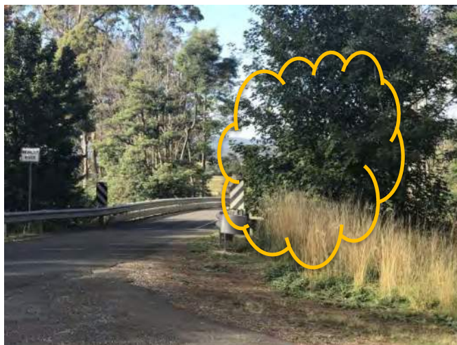
Figure 30 – Looking right along Porters Bridge Road from the Quarry access
