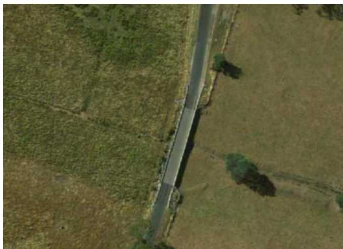
Figure 24 –Aerial view of Porters Bridge Road slab linked culvert.
