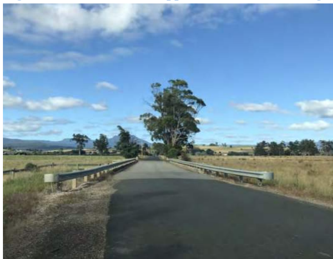
Figure 25 – South bound approach to Porters Bridge Rd slab linked culvert.
