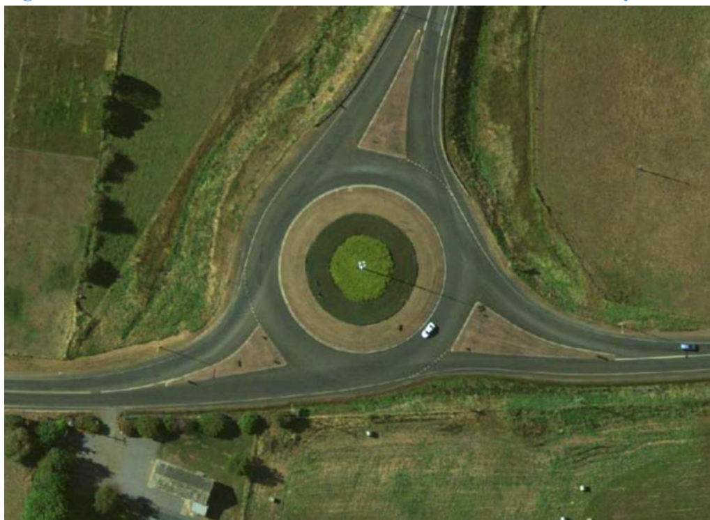
Figure 9 – Aerial view of Bowerbank roundabout with Meander Valley Road
