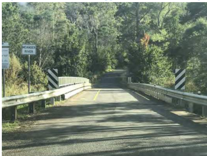
Figure 27 – North bound approach to Porters Bridge
