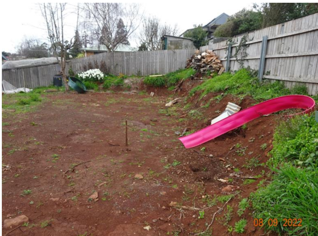
Figure 8: Photo showing the cut on site and the boundary fences.
