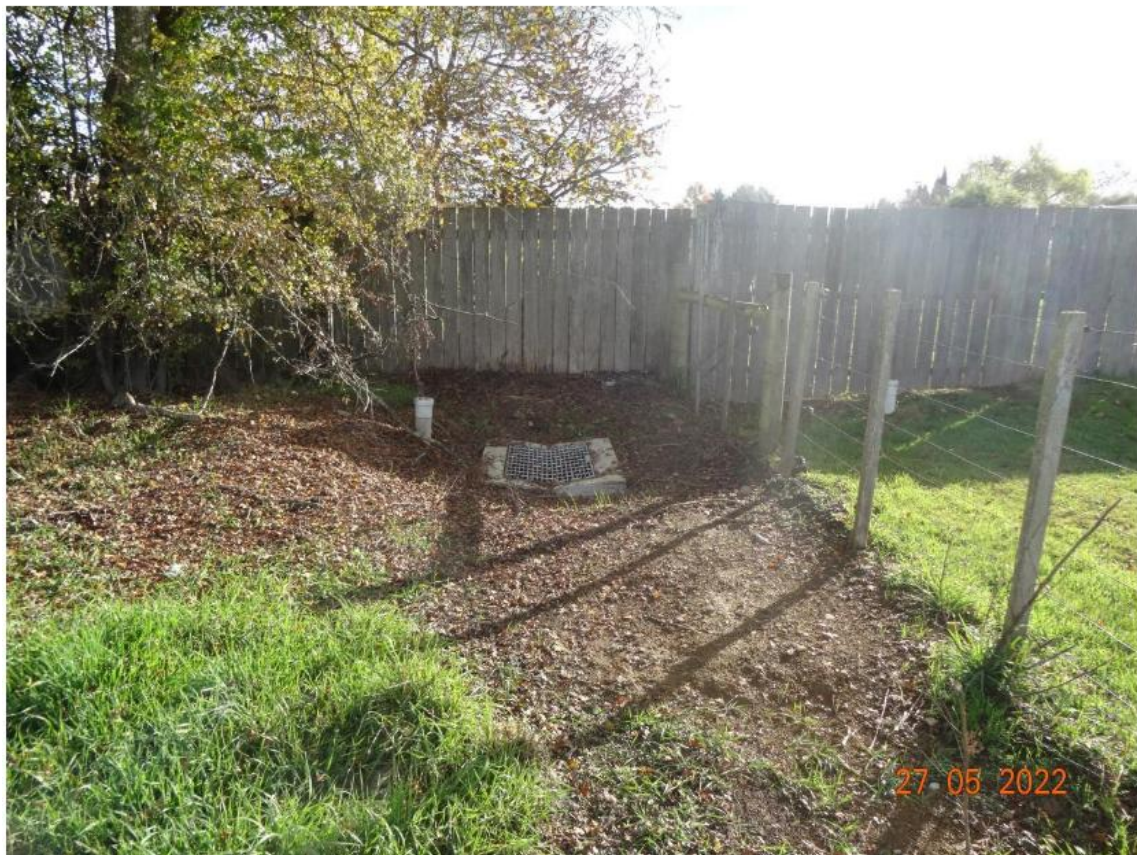
Figure 8: Stormwater connection located in the north-west corner.
