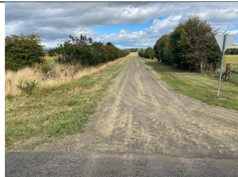
Figure 10 -Looking west along Pensioners Row subject site to the left.
