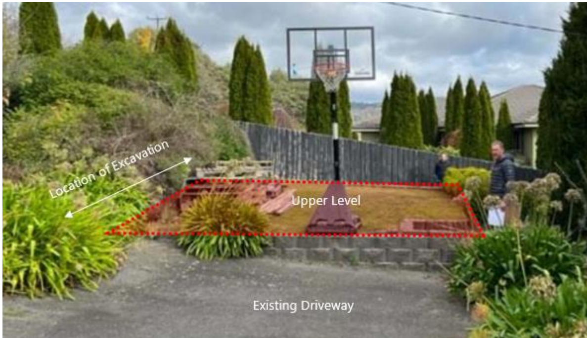
Figure 5: Upper level of the existing benched area.
