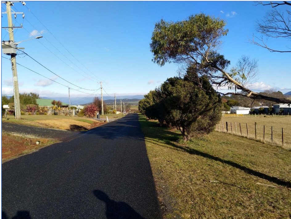
Image 12 – Looking west along Gleadow Street from proposed intersection to Emu Bay Rd intersection – measured sight distance is 205m.
