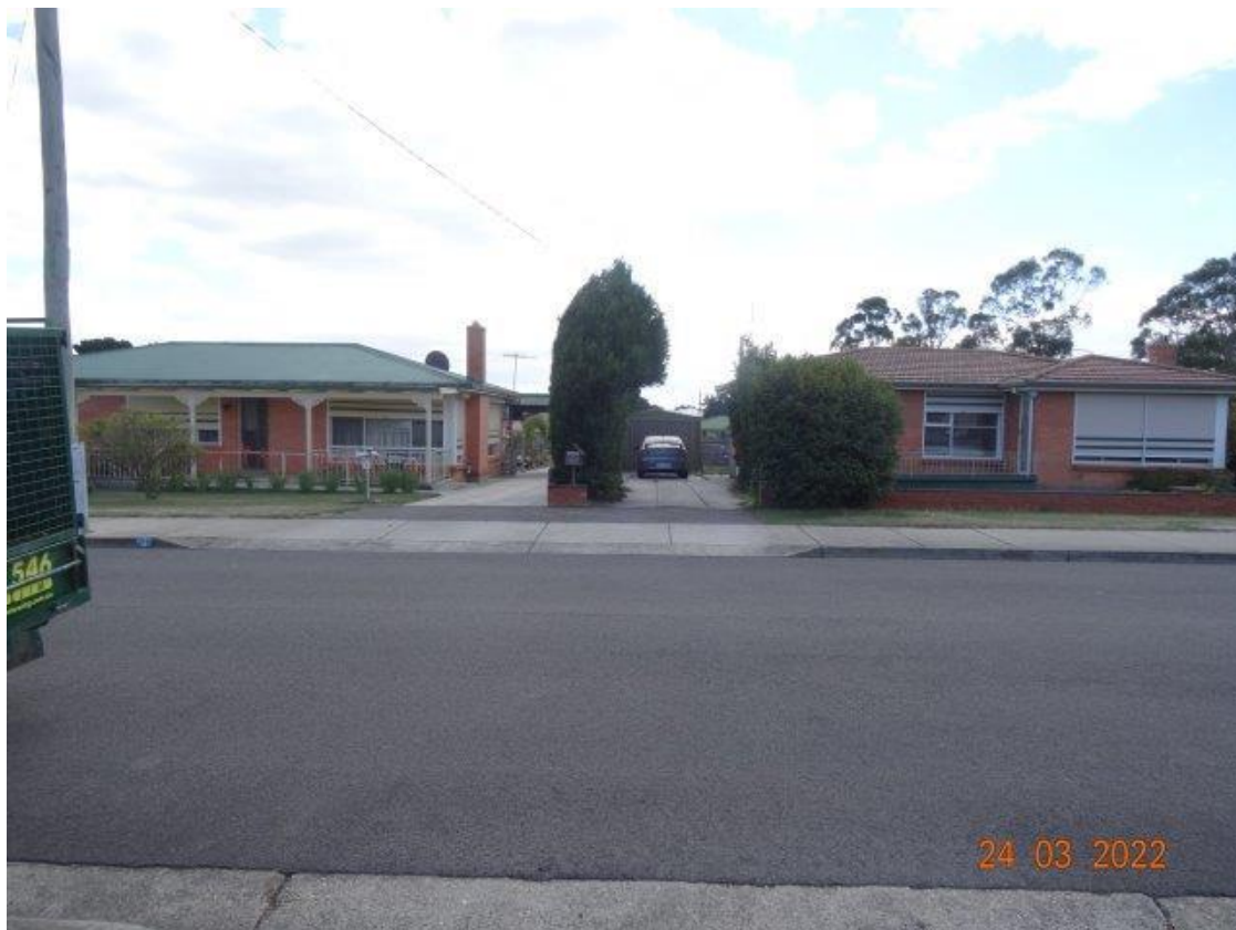
Figure 3: Photo of the existing dwellings located at 5 & 7 Bradford Avenue, Prospect Vale.
