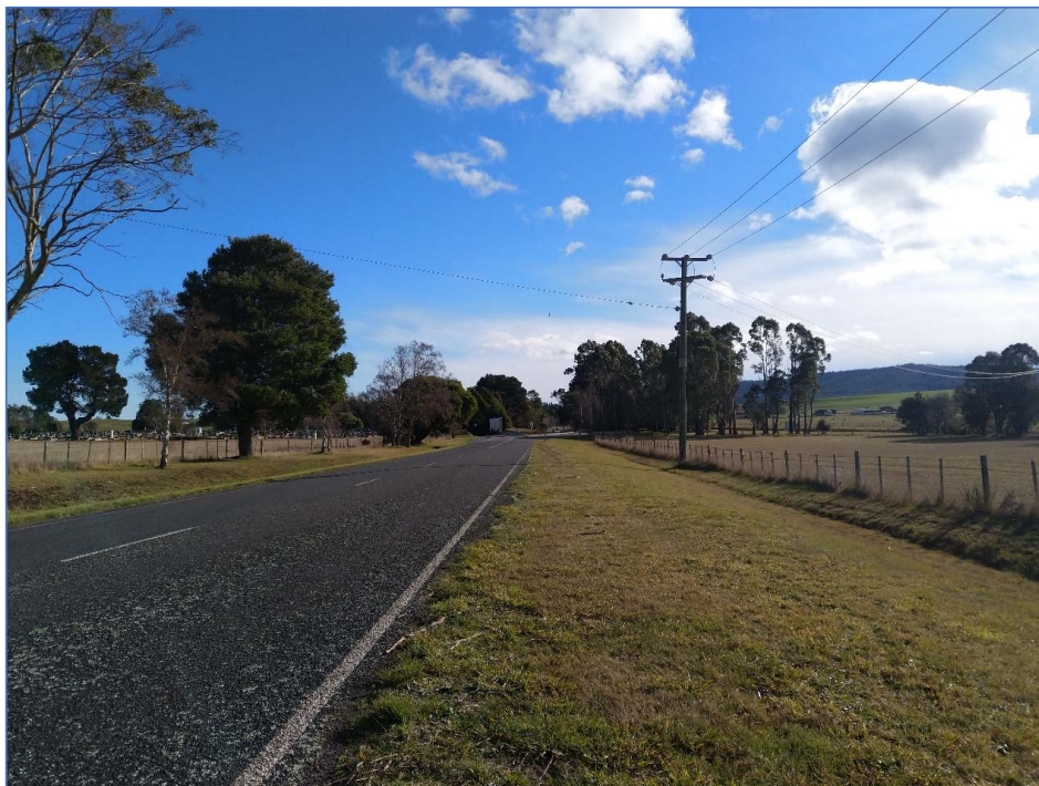
Image 11 – Looking north from proposed intersection to turning head and cemetery entrance on Emu Bay Road – measured sight distance is 195m.
