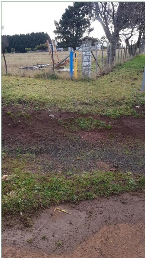
Figure A2-6: Existing hydrant on Emu Bay Rd
