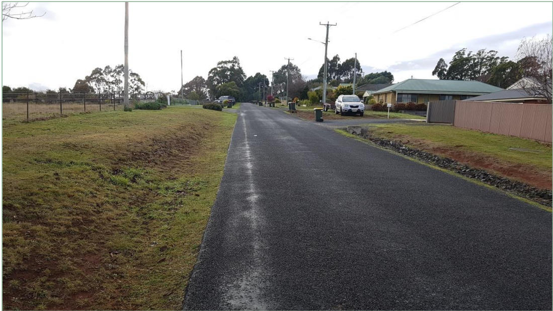
Figure A2-5: Gleadow St and the existing dwellings on the southern side.
