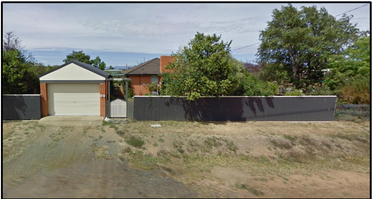
Photo 1: Existing residential dwelling to be contained on Lot 1.
