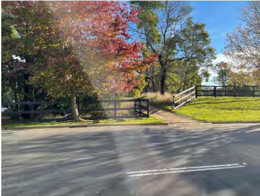
Photo 4 – Looking from Golf Course back towards open drain discharge, bio retention will be constructed on the rightside through the open gate.
