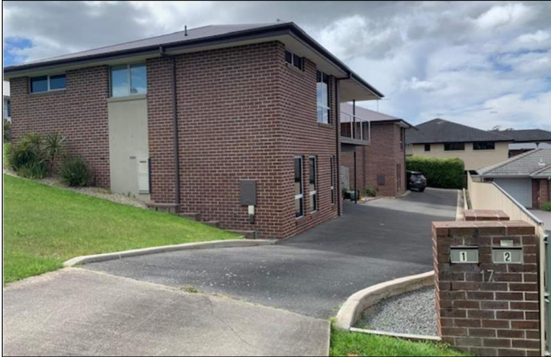
Photo 9: Existing south-western and south-eastern elevation of Unit 1. Unit 2 seen in the background. Looking from Bordin Street.
