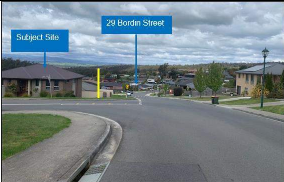
Photo 7: Streetscape of Bordin Street looking south-east. Yellow line indicates the extent of the proposed dwelling extension (excluding the deck).
