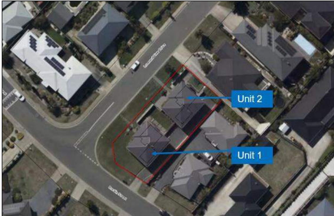
Photo 1: Aerial photograph of the subject site, outlined in red.
