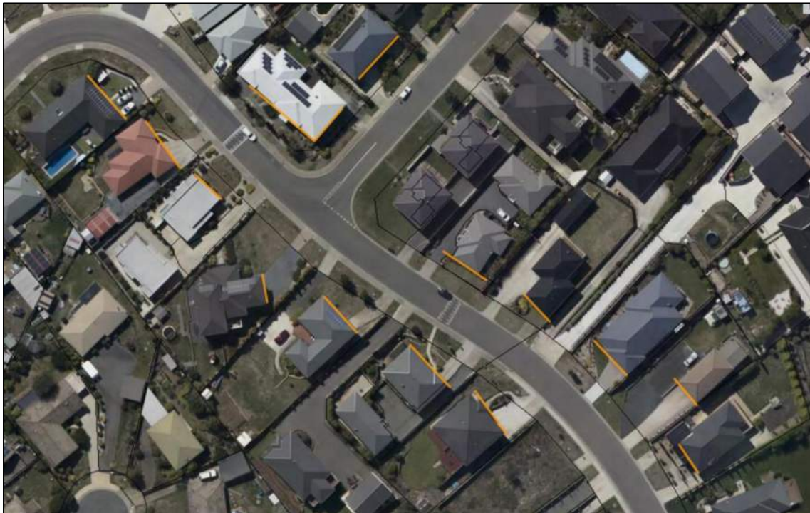
Photo 6: Established minimum setbacks of dwellings to the streetscape highlighted by the orange line.
