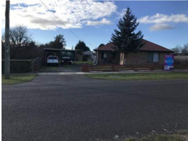
Figure 6 – Elevation view of access to 137 Dexter Street
