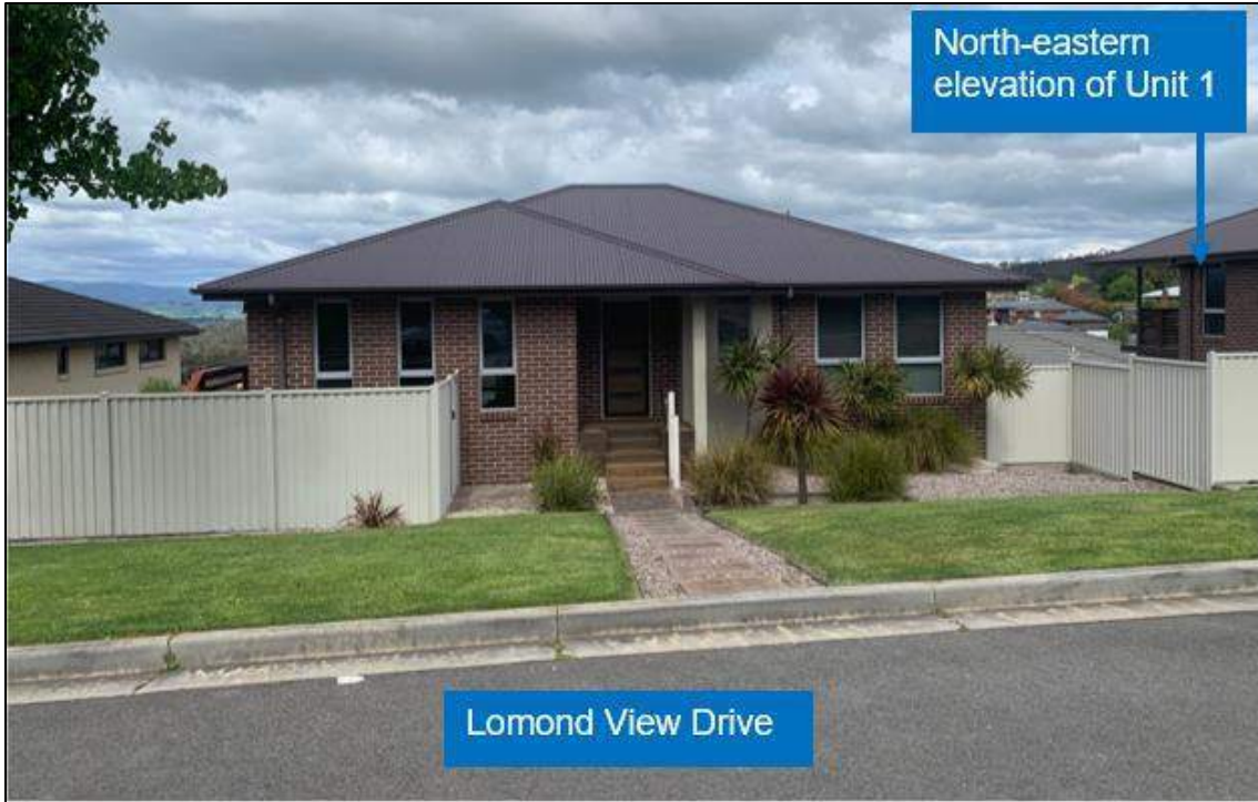
Photo 3: Unit 2, 17 Bordin Street, looking from Lomond View Drive towards the main facade and entrance of the dwelling.
