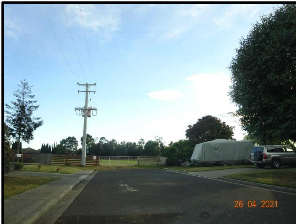
Photo 2: View towards frontage off Bimbimbi Avenue.
