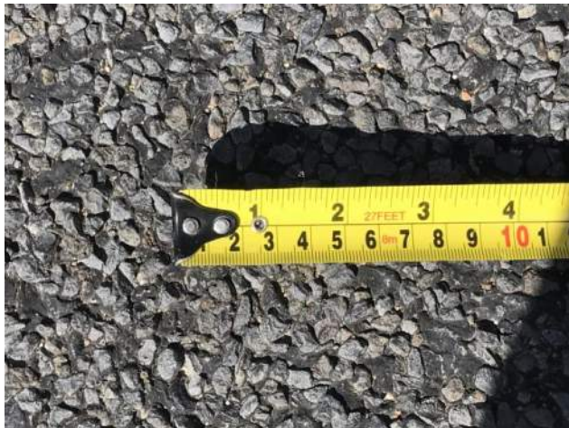
Figure 6 – Seal on Mole Creek Main Road
