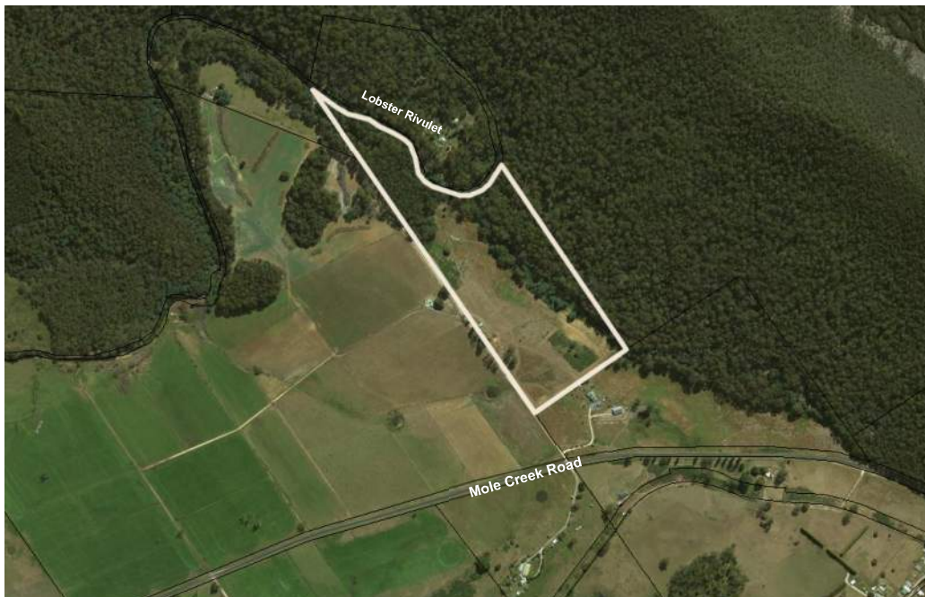
Figure 1 - aerial image showing the boundary of the site.
