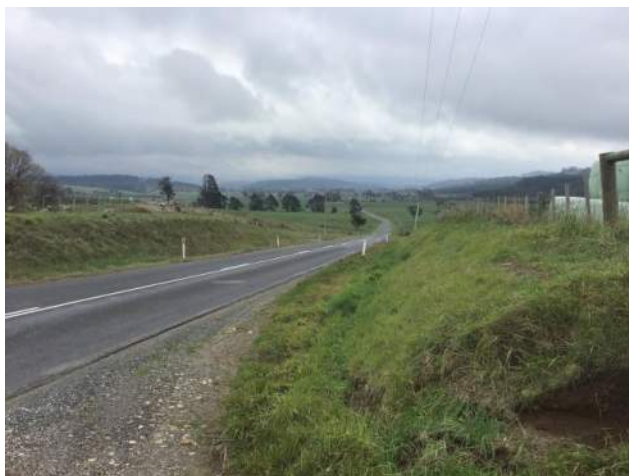
Figure 7 – Looking right along Mole Creek Main Road from the RoW road
