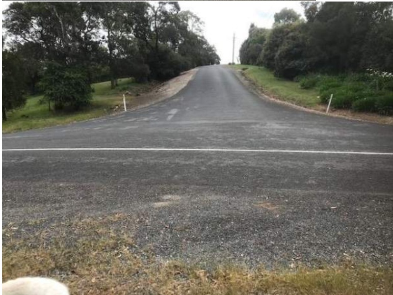
Canopus Dr and intersection with Zenith Court
