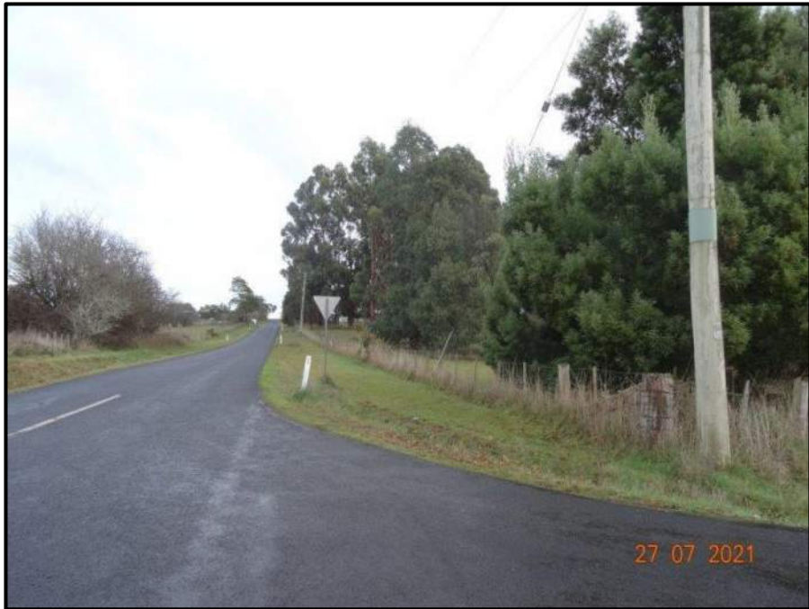
Photo 8: Looking west along Suburb Road showing the open drain to the right of the road.
