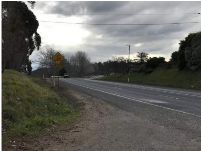
Figure A.15 – Looking left along Bass Hwy from Griffins Rd
