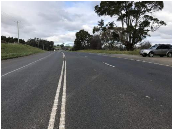
Figure A.17 – Bass Hwy Western approach to Griffins Rd
