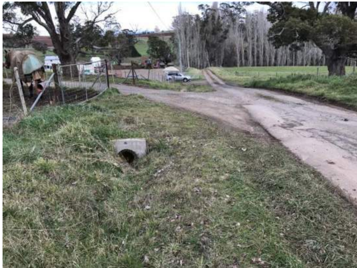
Figure A.9 – Culvert with headwalls at dwelling access
