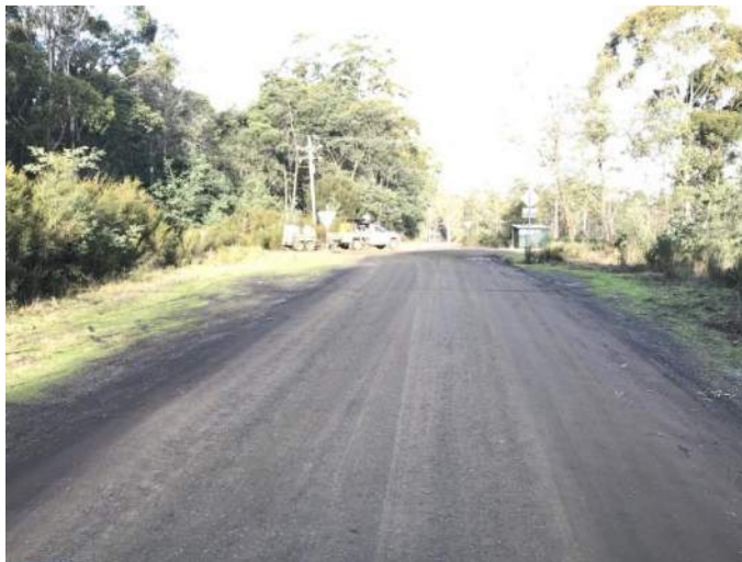
Figure 6 – Wadleys Road Northern approach to River Road intersection
