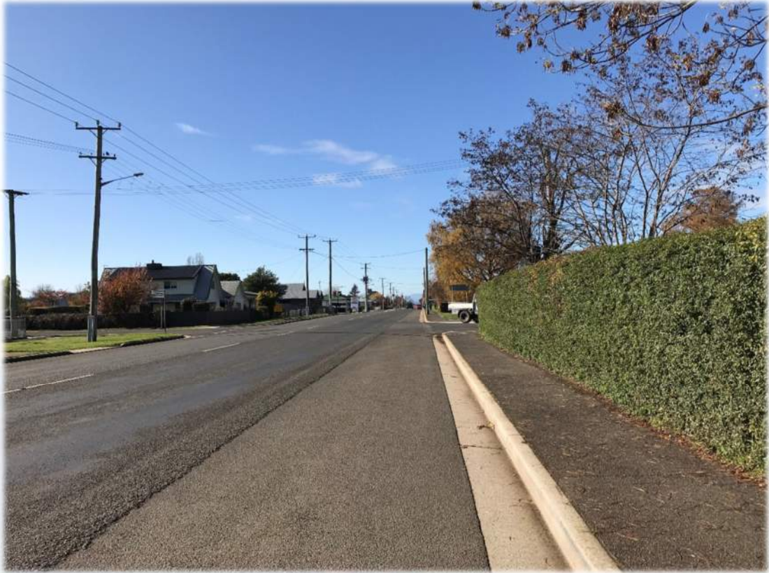
Figure 7 – Lot A: looking right from access location
