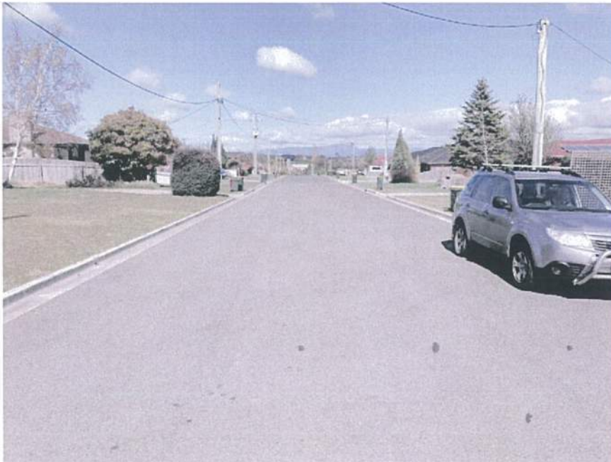
Figure 5 Looking west along Scott Street towards Bartley Street Junction
