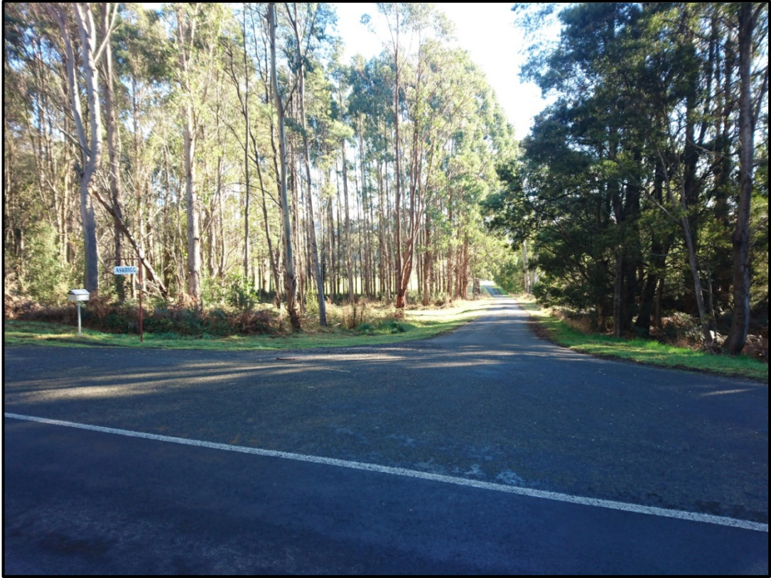
Figure 2: access to subject road off Mole Creek Road (looking north)
