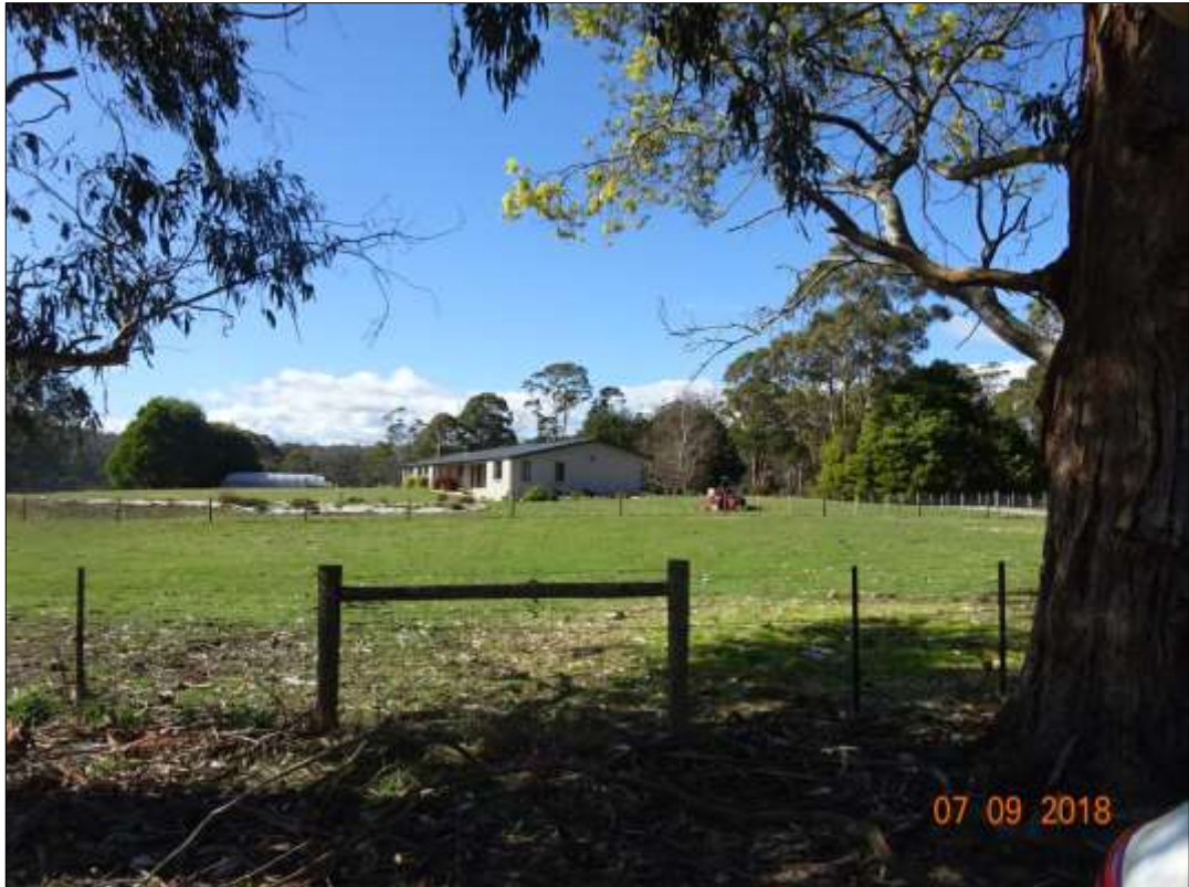
Photo 2: dwelling at 180 Wandilla Road, viewed from east boundary
