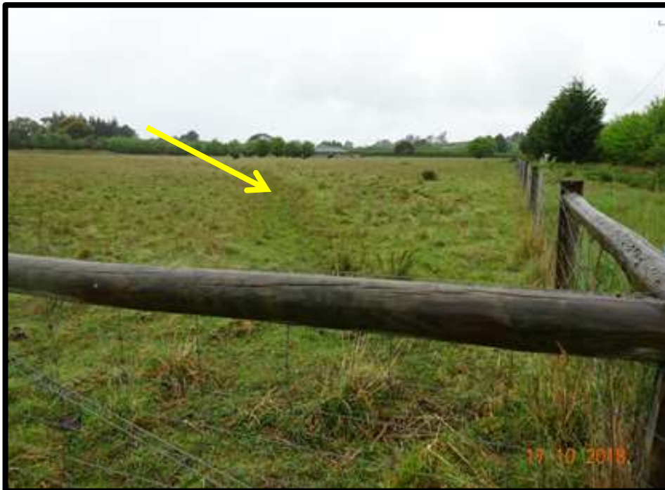
Photo 4: showing shallow open drain at south-west corner of land
