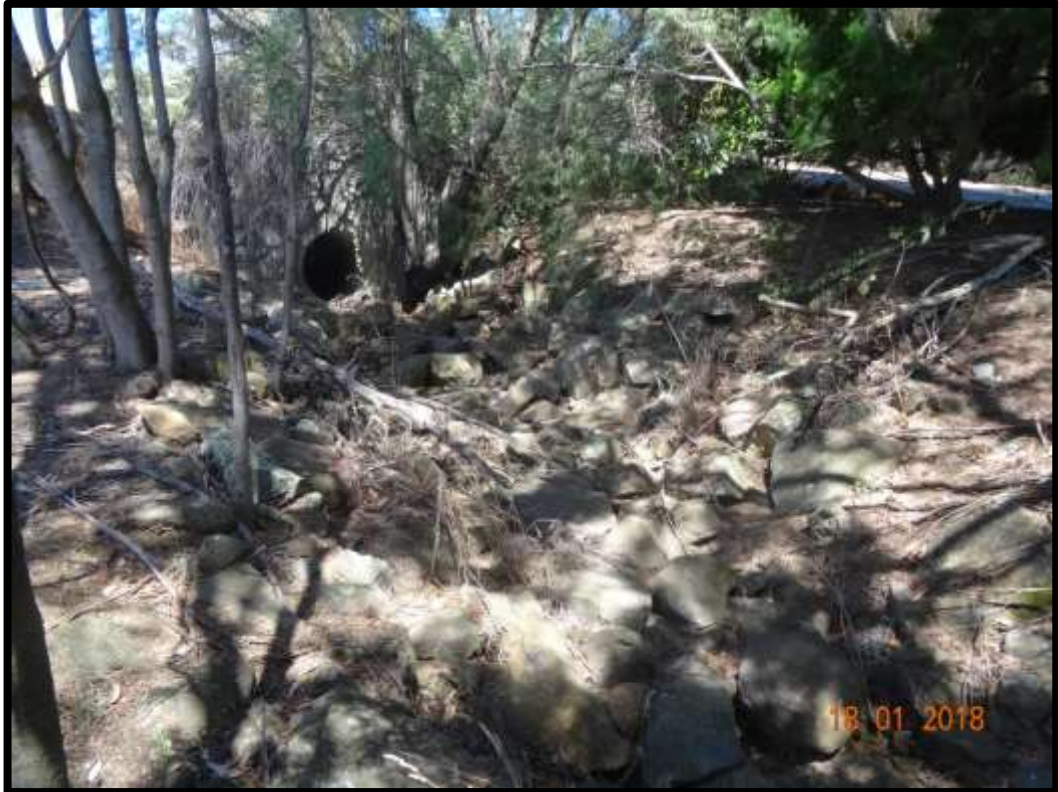
Photo 4: view of open drain
