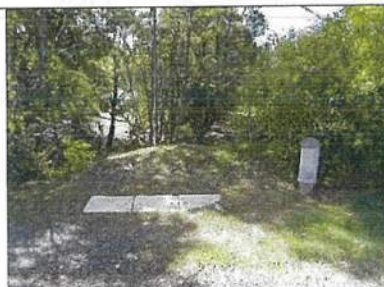
Figure 4 - Telstra Pit and Pole.
