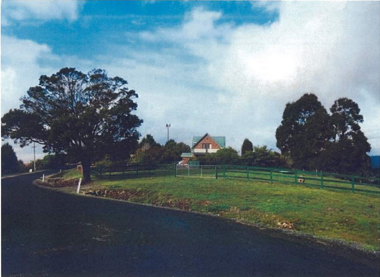
Figure 15 – Indicative view from Zenith Court, approximately 270m north-west from the proposed site. Please note that this is showing a tower height of 30m rather than 25m.
