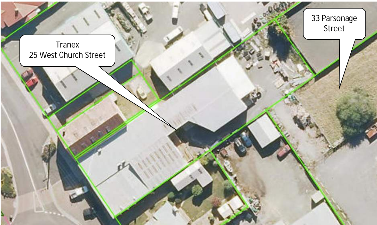
Figure 2 - Aerial Photograph of Tranex (from theList)
