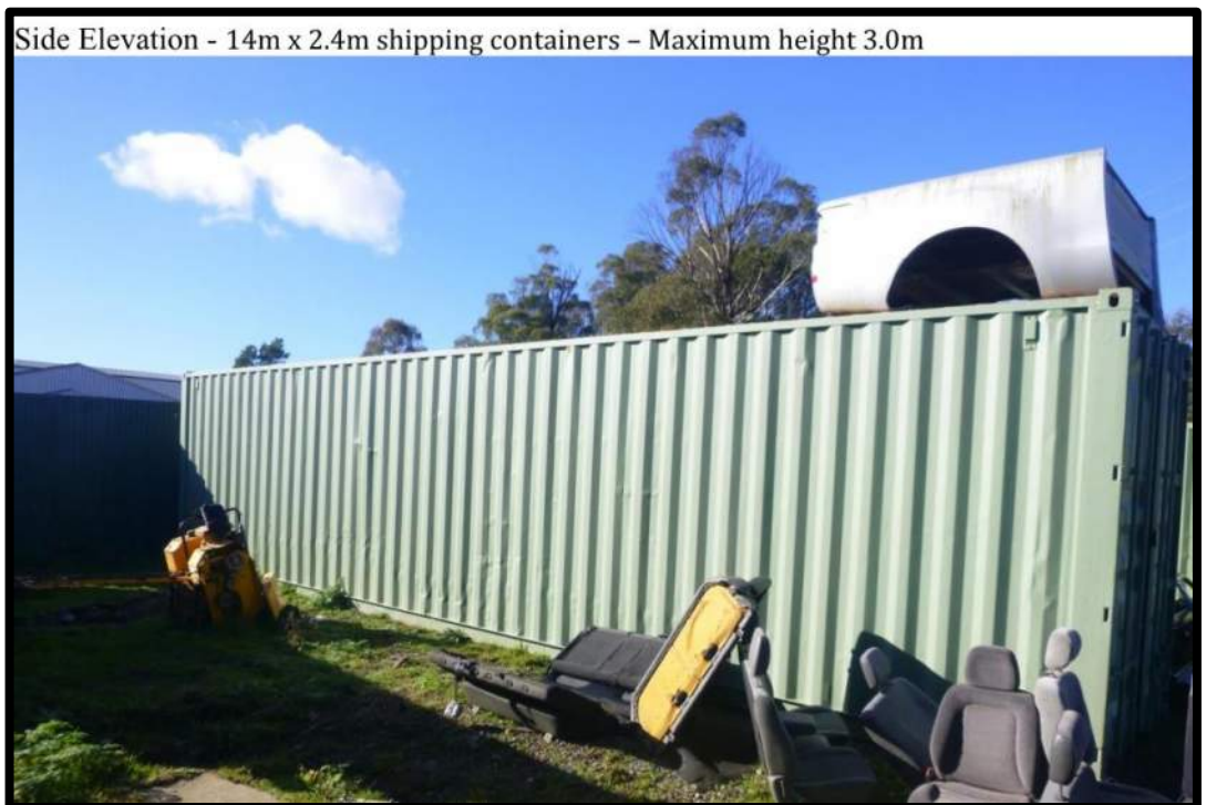
Figure 3: side elevations provided by the applicant and typical of the proposed 14m shipping containers identified as No.1 in Figure 2 above
