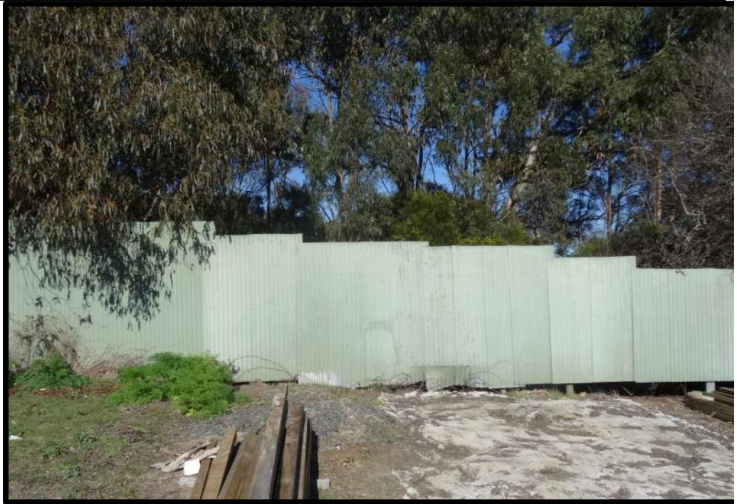
Photo 9: Existing screen and vegetation to the south-west of buildings 4 and 5
