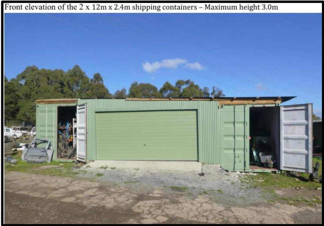
Figure 4: front elevations of storage building identified as No.2 in Figure 2 above, provided by the applicant
