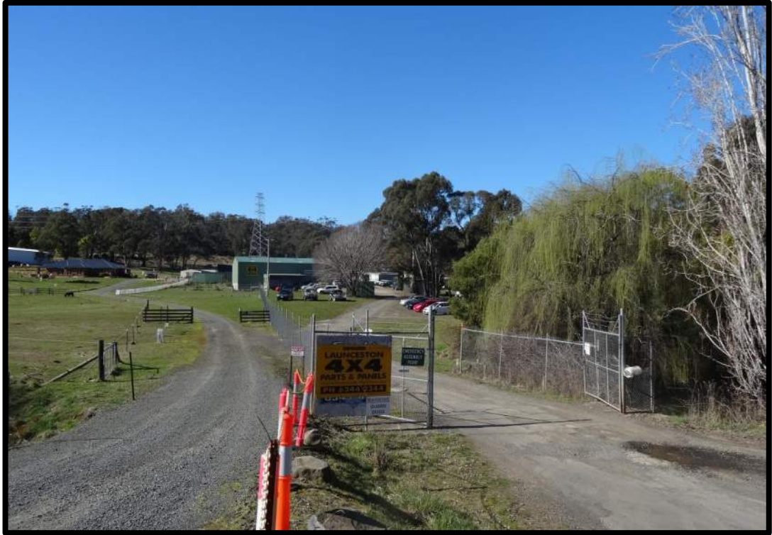
Photo 1: subject title, looking south-east from the access on Meander Valley Road
