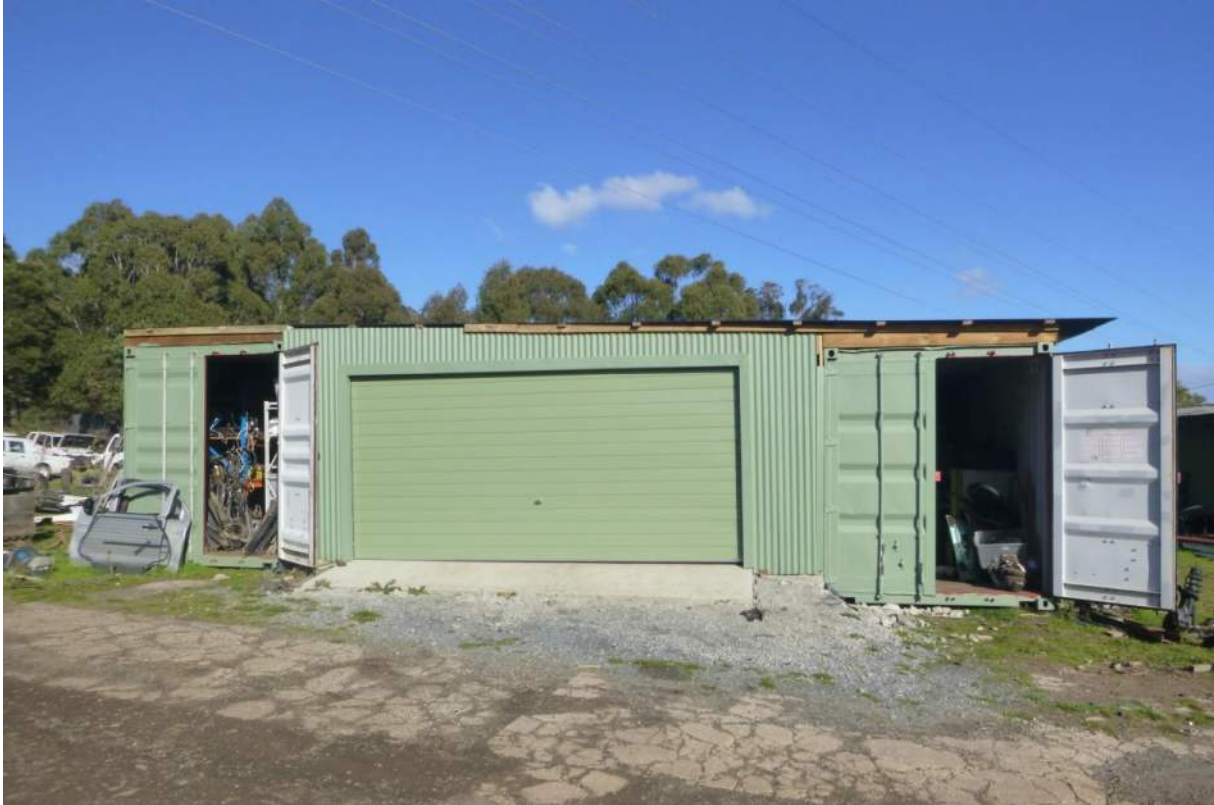
Front elevation of the 2 x 12m x 2.4m shipping containers – Maximum height 3.0m
