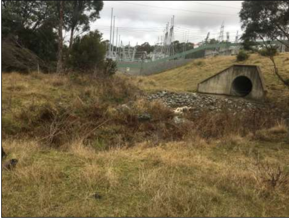
Figure 8 – WP 130; North-western discharge point (north of substation)
