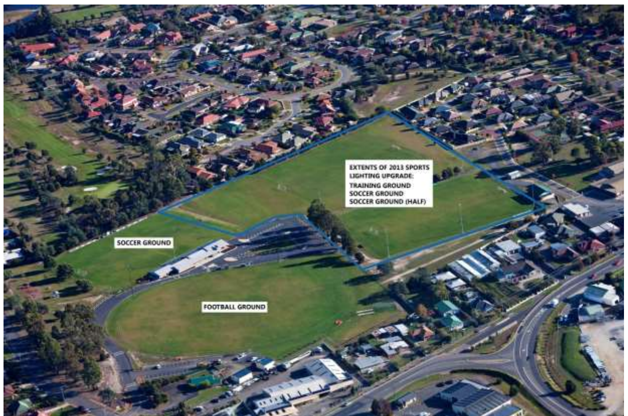
Image 1: Showing the location of the football and soccer grounds and extents of 2013 sport lighting upgrade at Prospect Vale Park.
