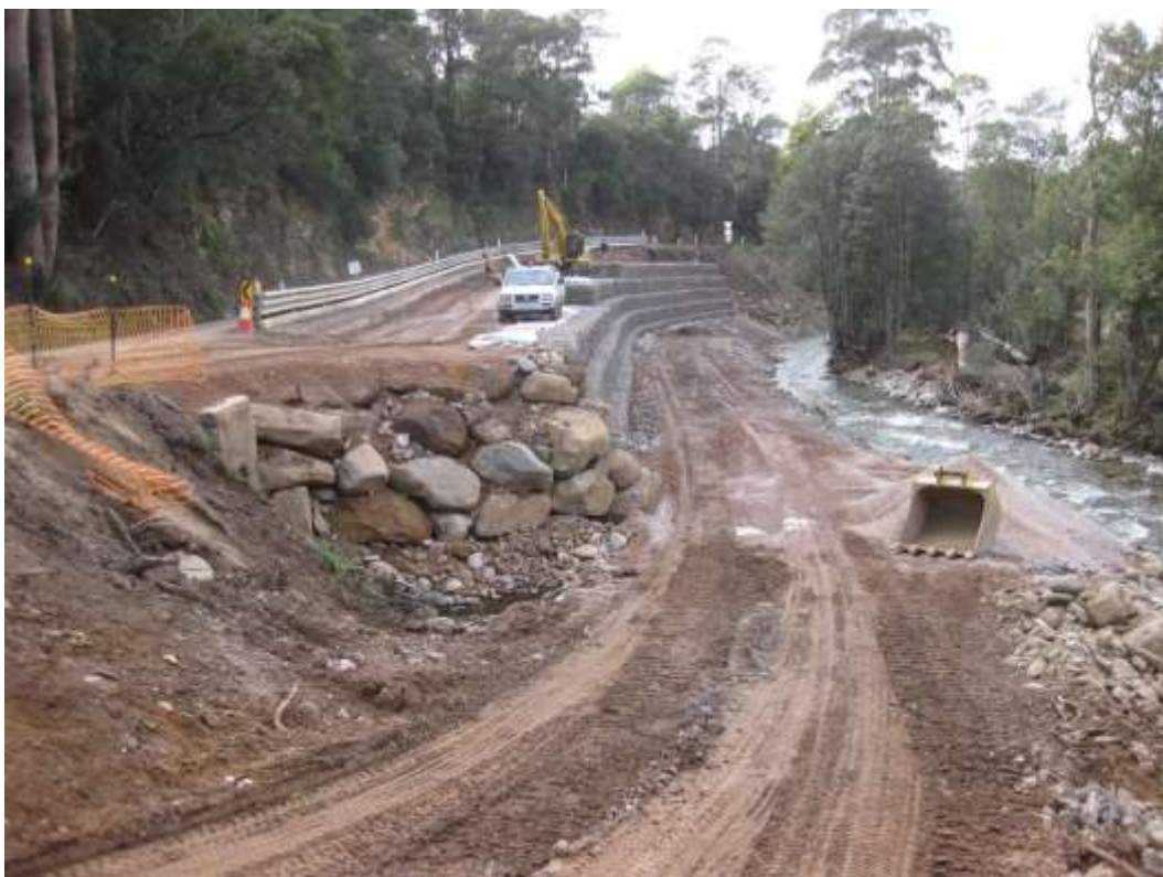
Photo 2: Gulf Road embankment reconstruction
