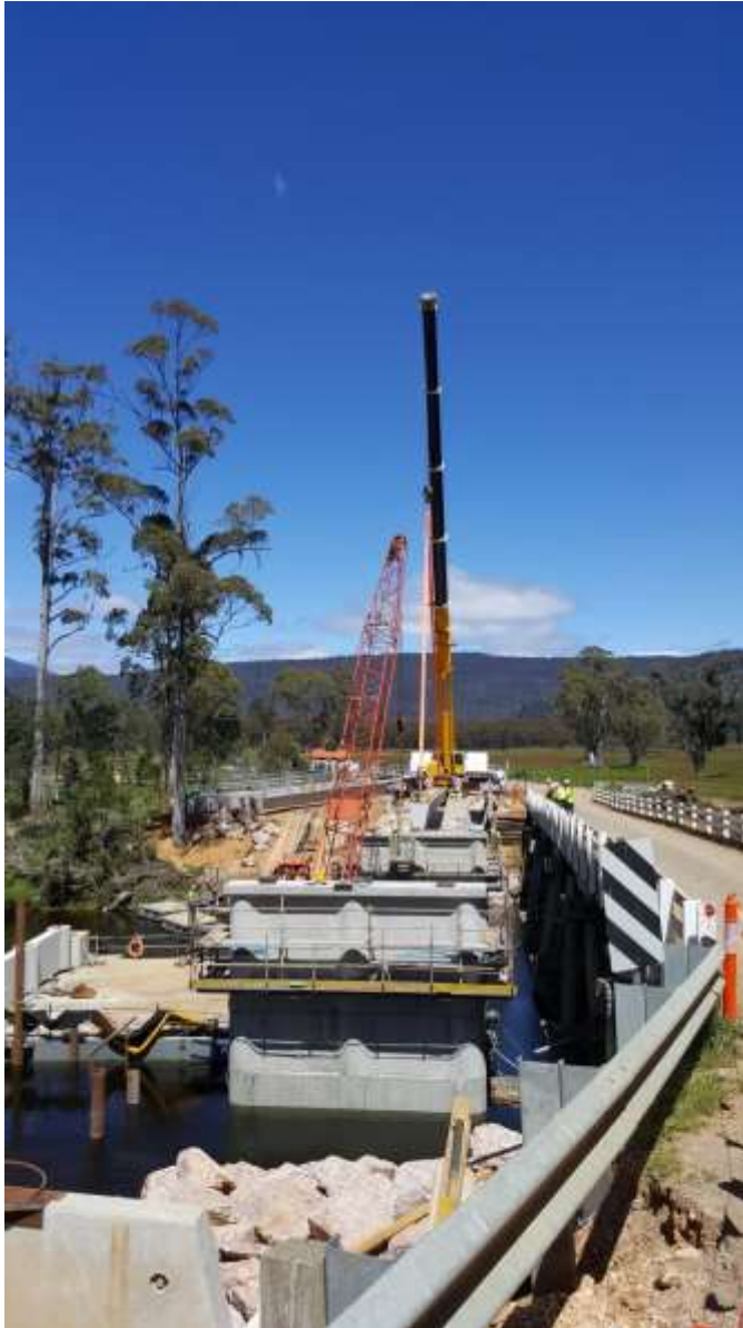
Photo 1: Union Bridge Road bridge reconstruction
