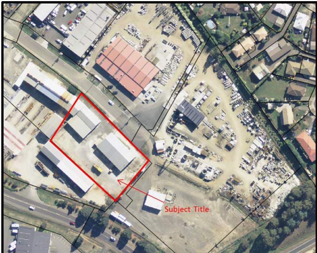
Photo 1: Aerial photo of subject title and surrounding land.
