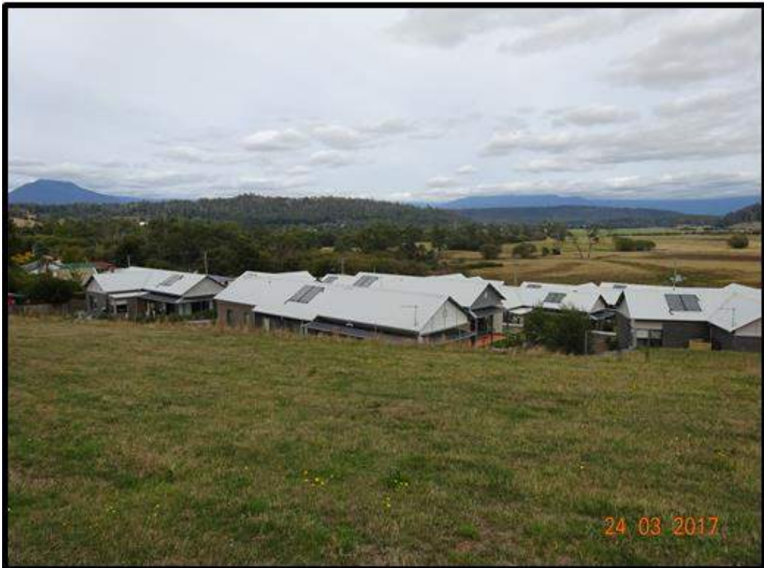
Photo 2: Existing multiple dwellings at 35 Moriarty Street, viewed from within the subject title.
