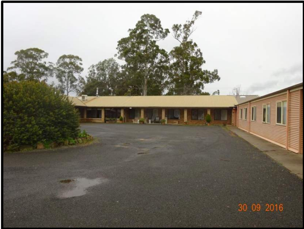
Photo 3: Existing accommodation complex, looking east from the internal driveway
