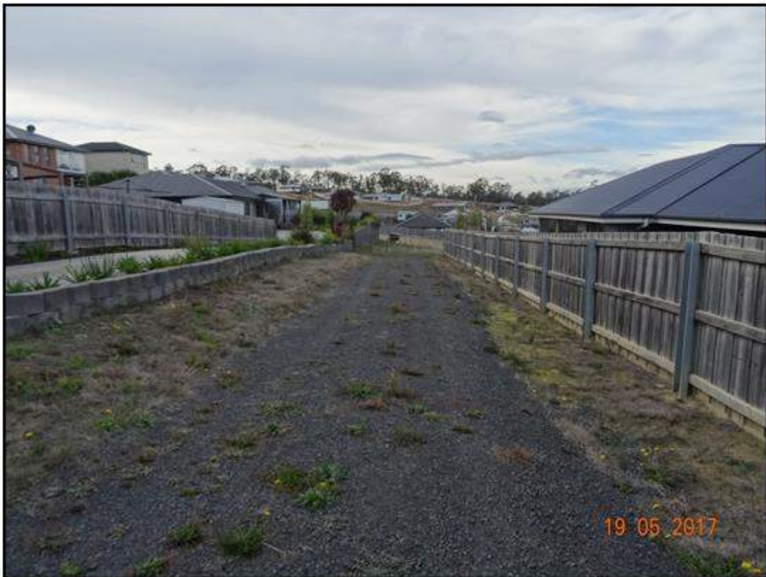
Photo 4: Internal access to site
