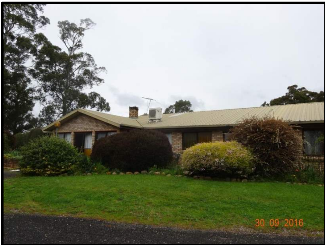
Photo 4: Existing accommodation complex, looking south from the internal driveway
