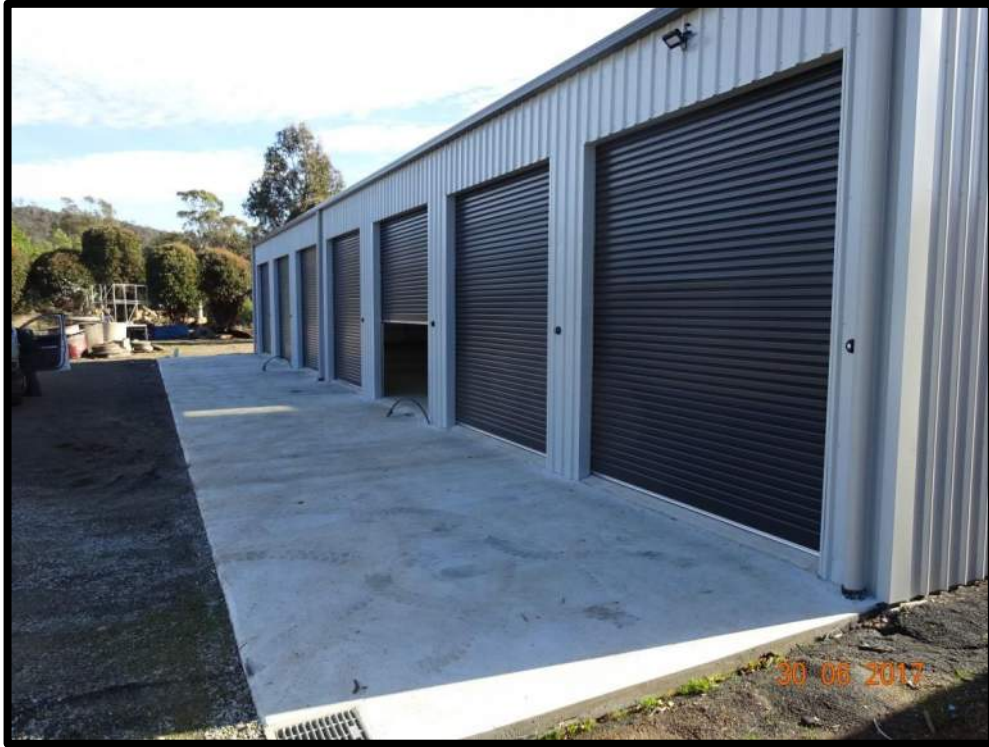
Photo 1: south-west view of subject building
