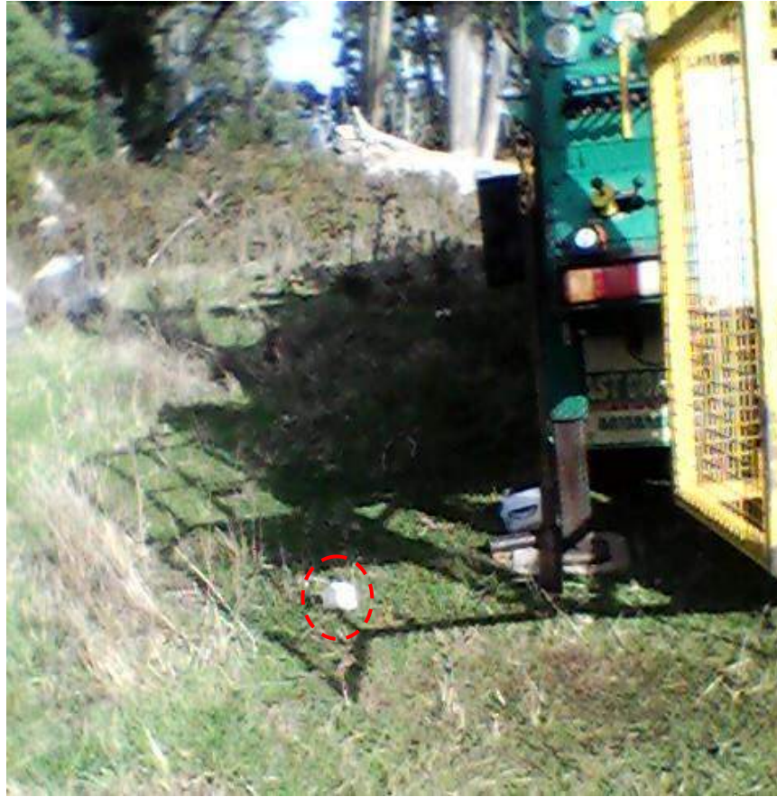
Photo 1. Drilling rig set up adjacent to centre peg
