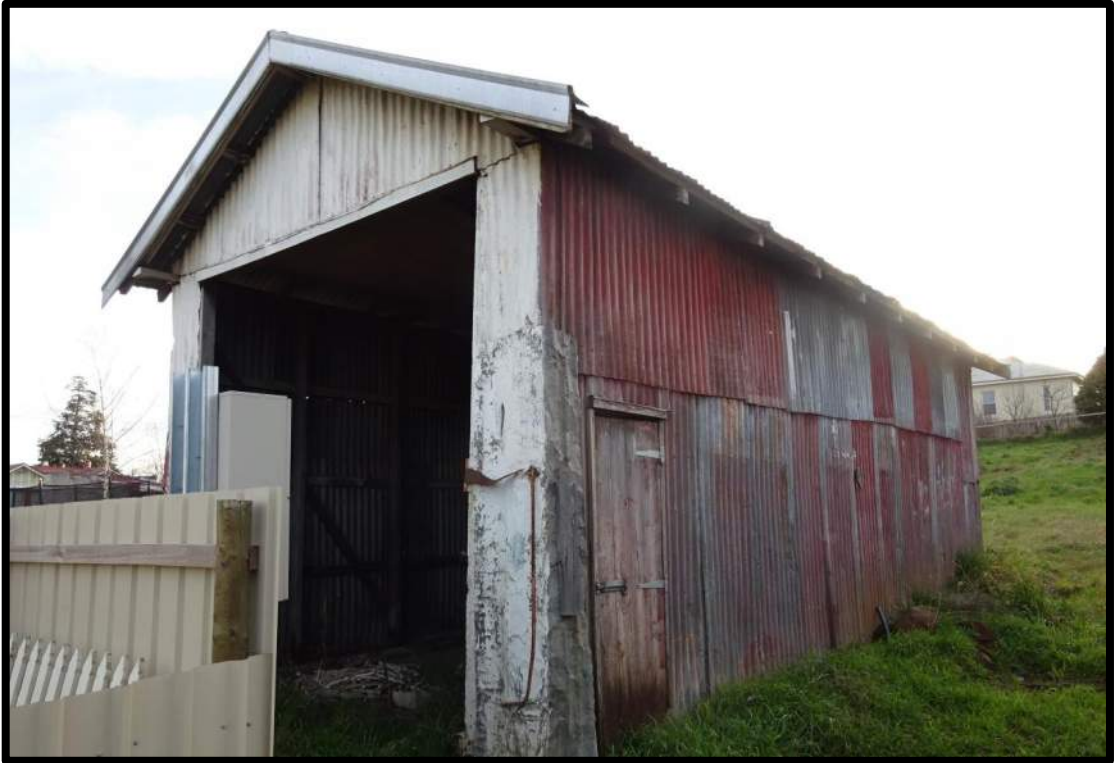
Photo 2: Existing outbuilding at 45A Parsonage Street, to be demolished
