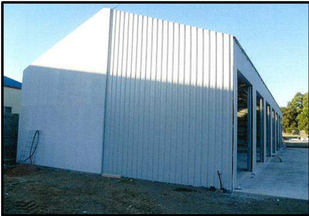
Photo 2: north-east view of subject building
