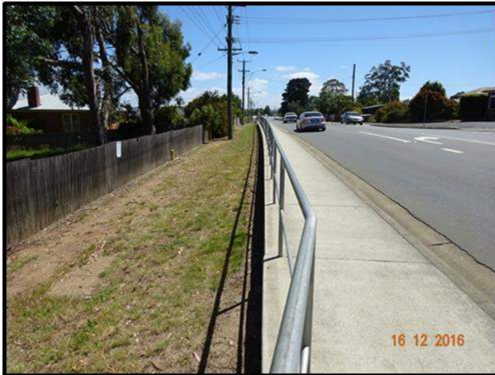
Photo 7: looking north along Westbury Road
