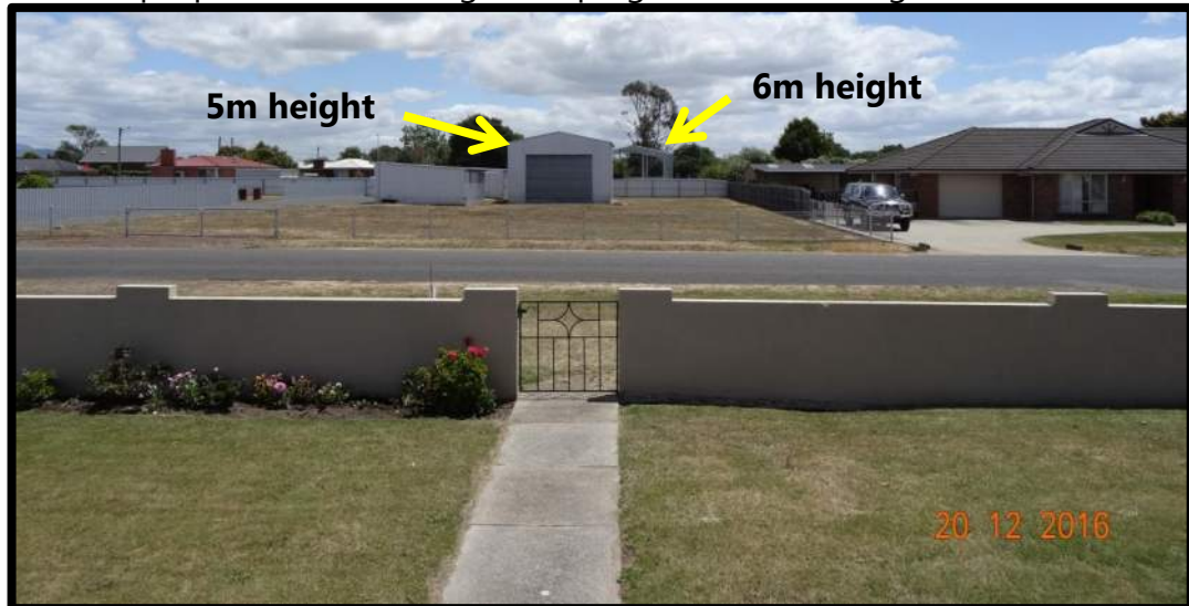
Photo 7: view from 29 East Street looking west, showing overall height of outbuildings
