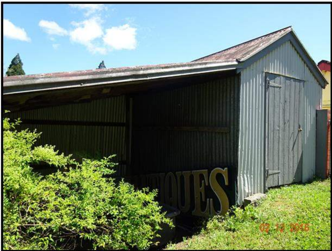
Photo 4: outbuilding proposed to be demolished
