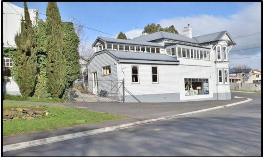
Photo 2: proposed Lot 2, viewed from East Parade, showing the existing dwelling, shopfront and outbuilding
