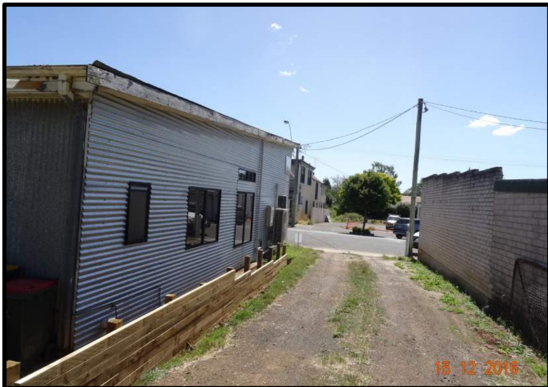
Photo 3: existing access viewed from within the property
