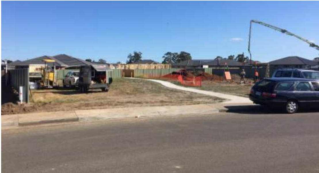
Image 7 - Bordin Street property with play equipment and landscaping under construction.
