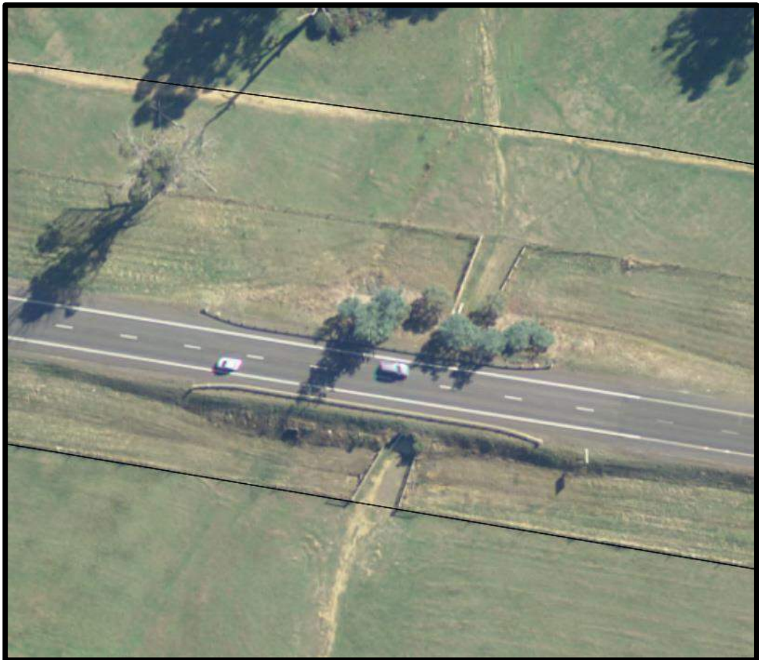
Photo 6: Aerial view of existing stock underpass, connecting the land to the north and south of the Bass Highway
