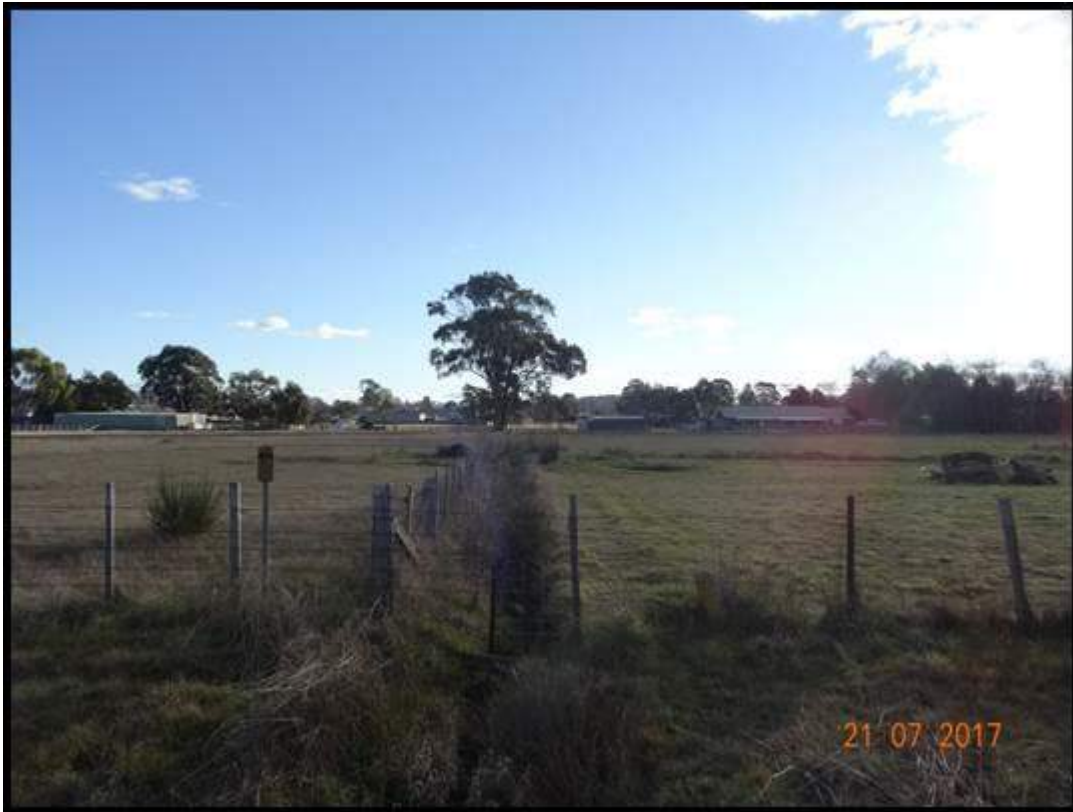
Photo 7: Existing public drain crossing 12 Pensioners Row
