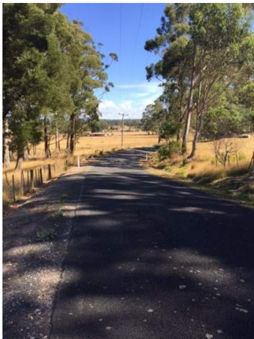
Figure 6 – Road looking West
