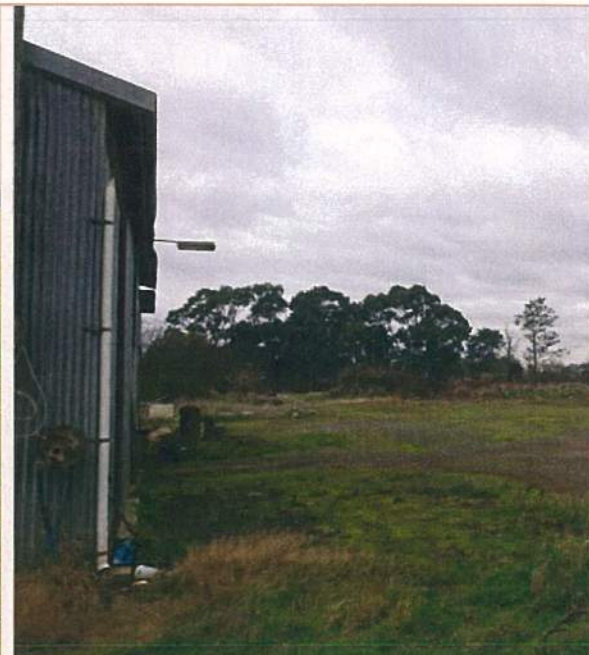
View looking southeast towards Lot 1
