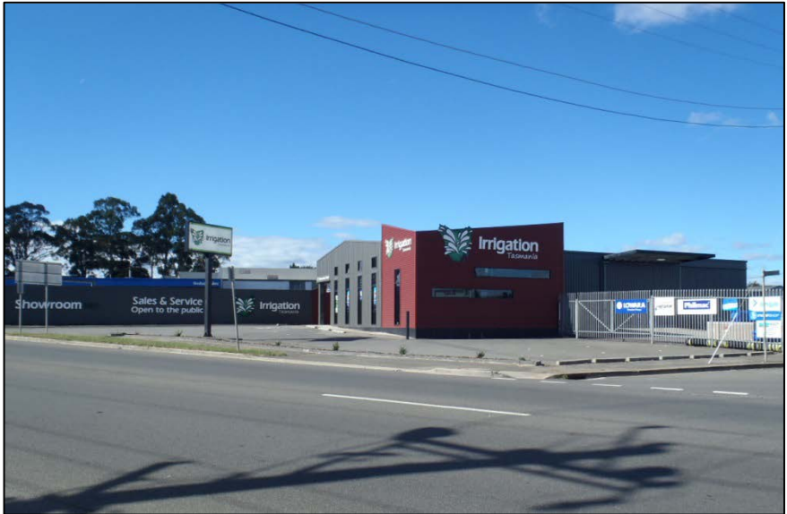
Photo 5 – Irrigation Tasmania 379-381 Westbury Road, corner Donald's Avenue.
