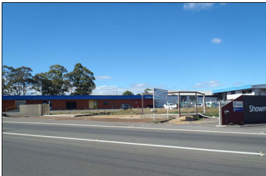
Photo 4 – Partially demolished site – 375-377 Westbury Road
