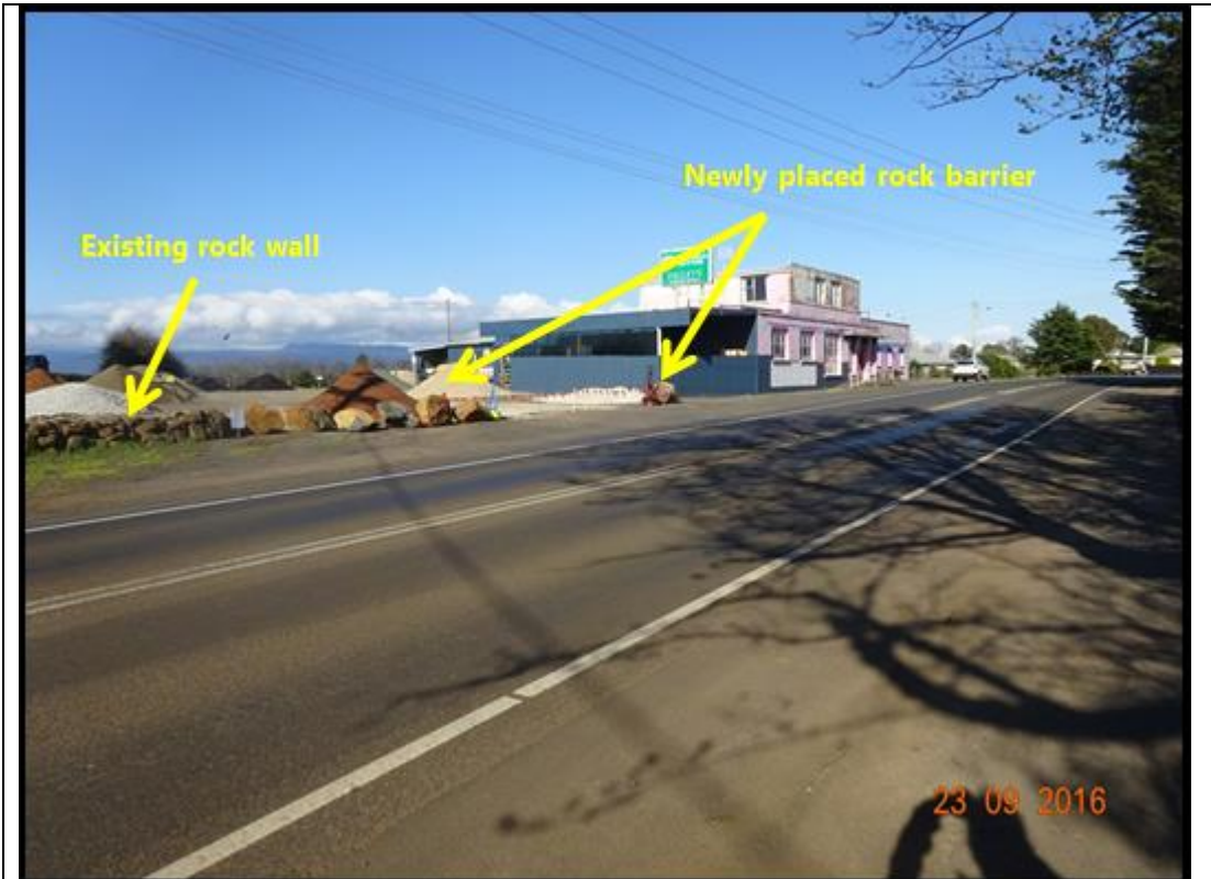
Photo 6: showing existing rock wall and newly placed large rock barrier
