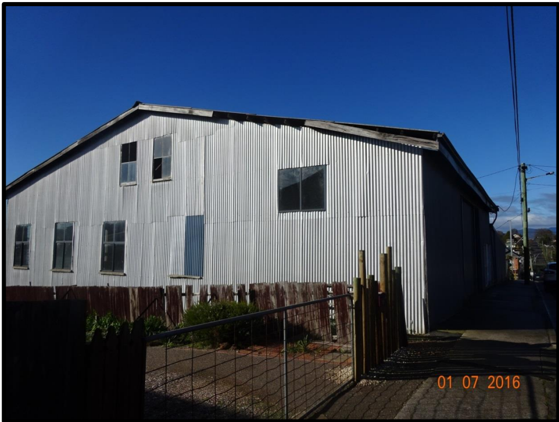
Photo 4: Existing building viewed from West Barrack Street looking south-east
