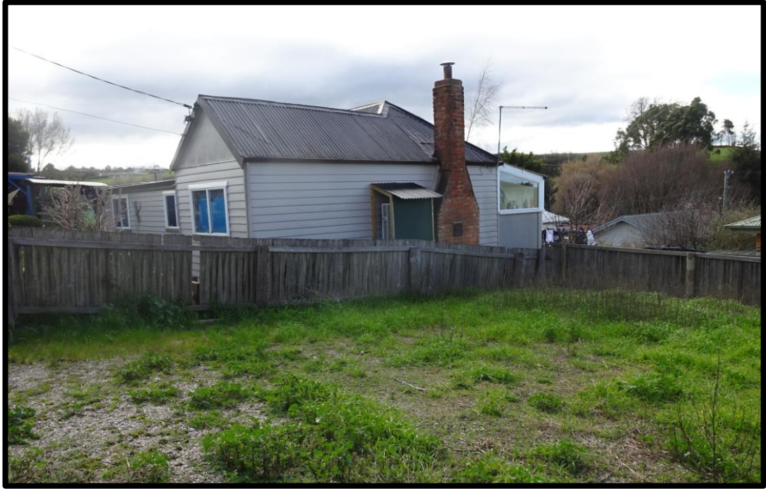
Photo 7: Adjoining residence at 13 West Barrack Street
