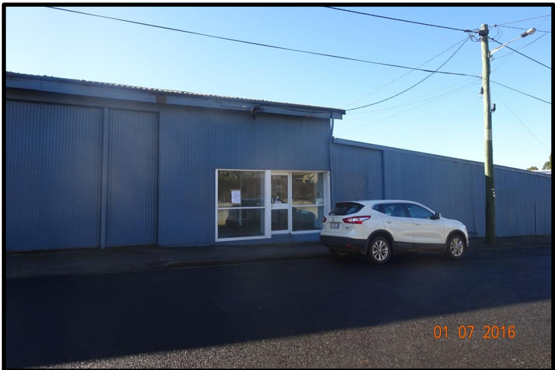
Photo 2: Subject property and existing buildings viewed from West Barrack Street
