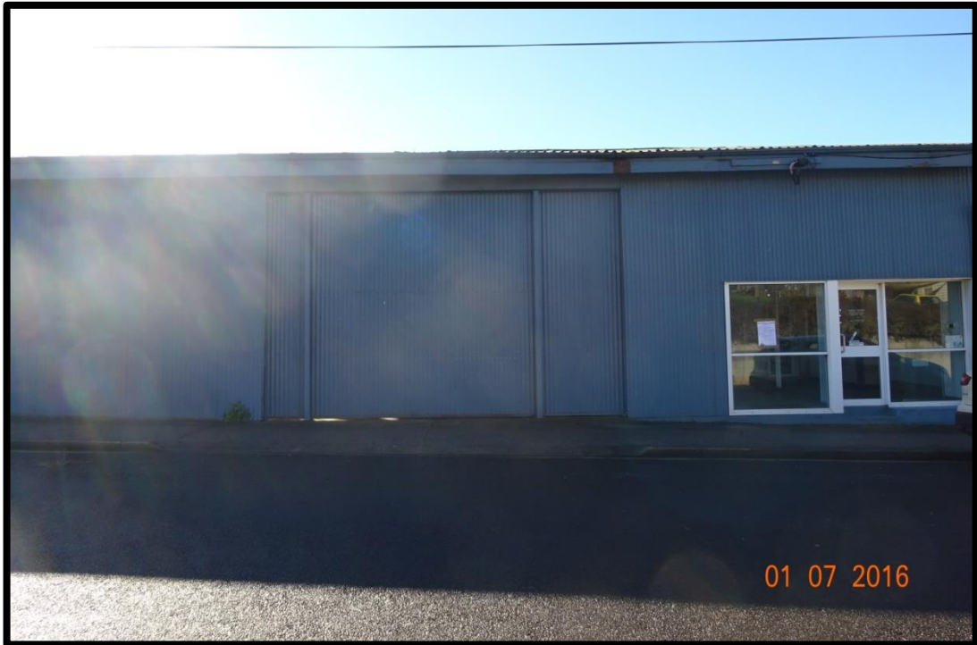
Photo 3: Existing buildings viewed from West Barrack Street looking north-east
