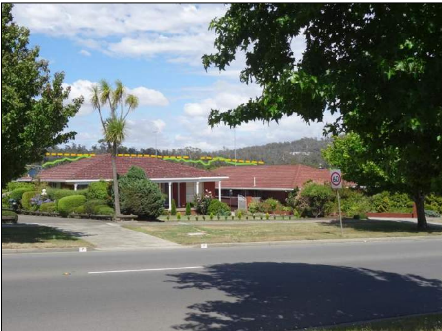
Photo 14 – View to the western end from Country Club Avenue.
