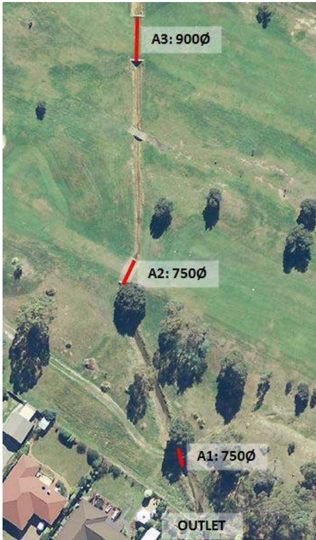
Figure 15. Eastern drain culverts
