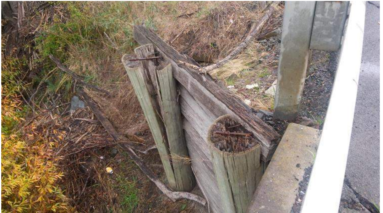
Photo 2: Eastern downstream abutment wingwall
