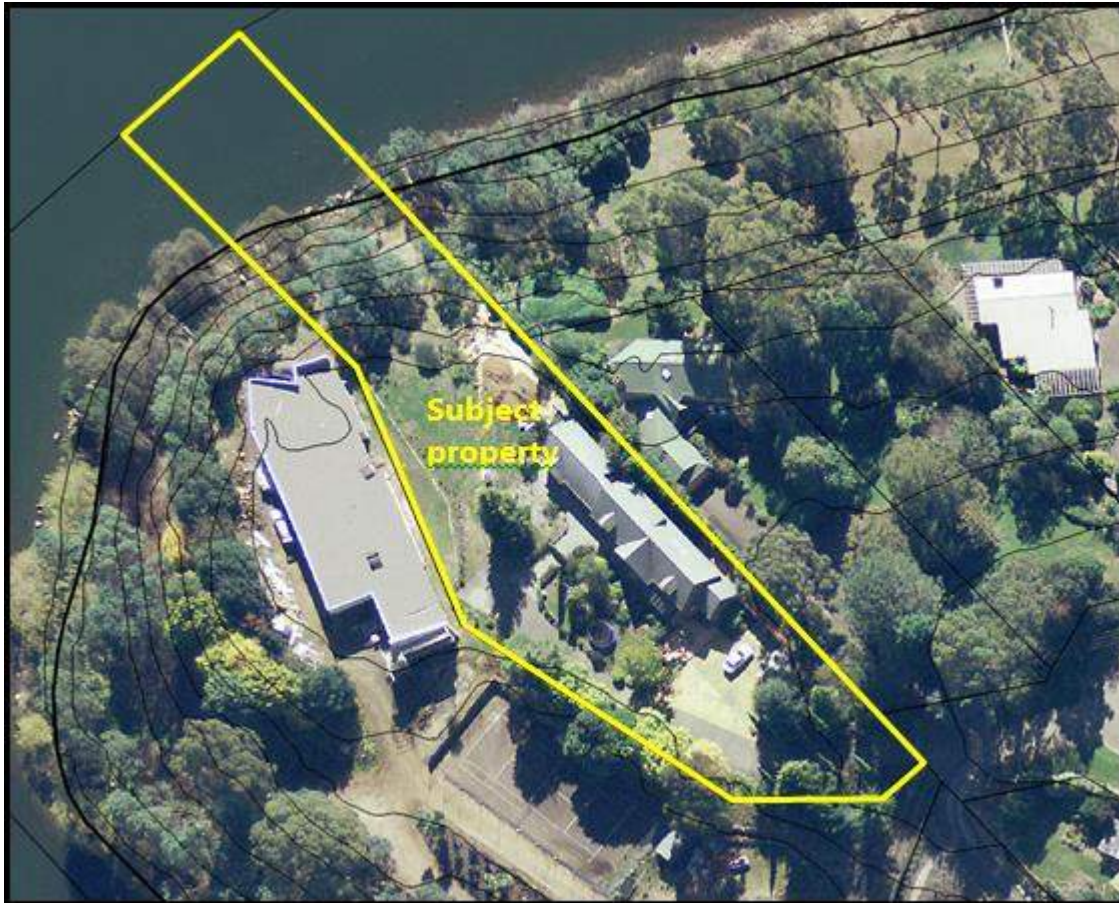
Photo 2: Aerial photo with 2m contours internal shown.
