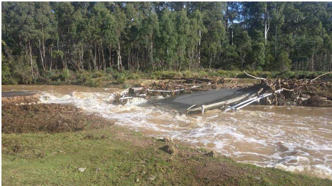
Photo 1 – Union Bridge Road
