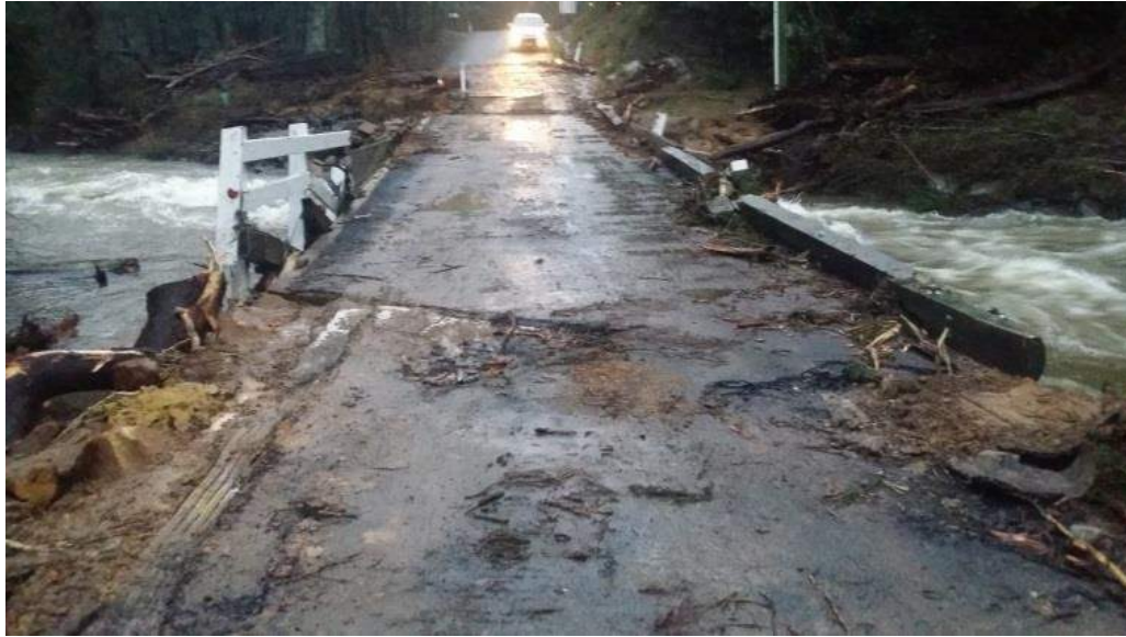
Photo 6 – Gulf Road, Liffey
