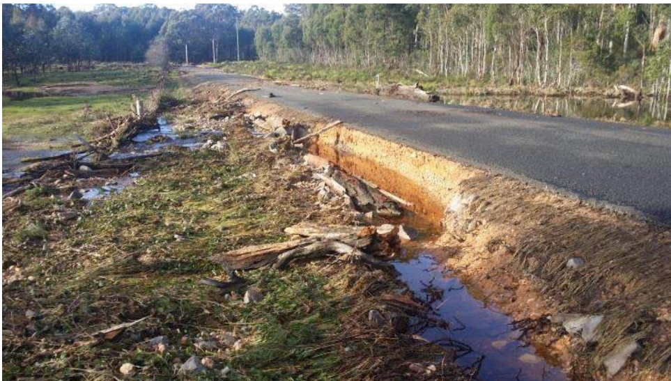
Photo 11 – Union Bridge Road
