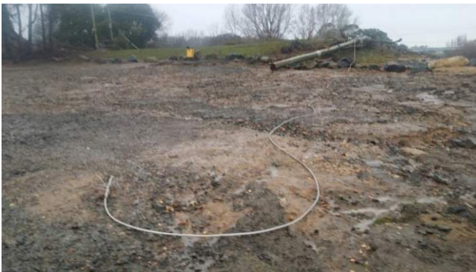
Photo 13 – Hadspen Boat Ramp
