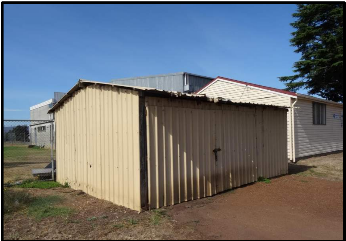
Photo 3: Storage building to be demolished.
