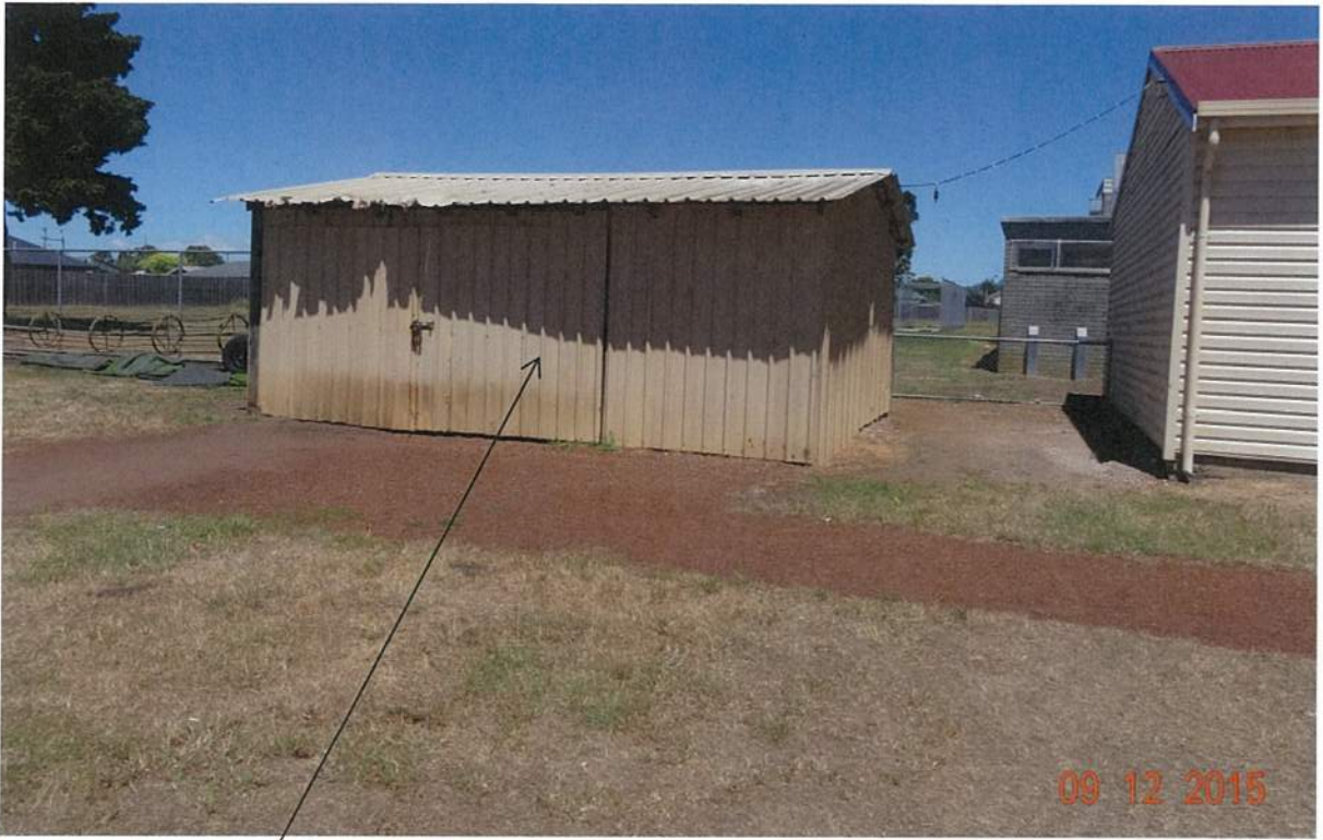
Outbuilding to be demolished.
