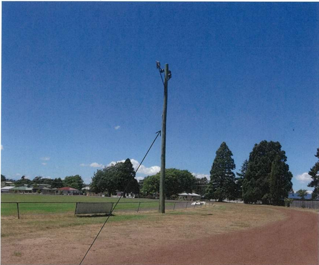
Light pole to be relocated.
