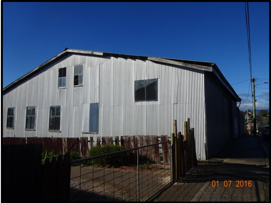
Photo 4: Existing buildings, viewed from West Barrack Street, looking south-east.
