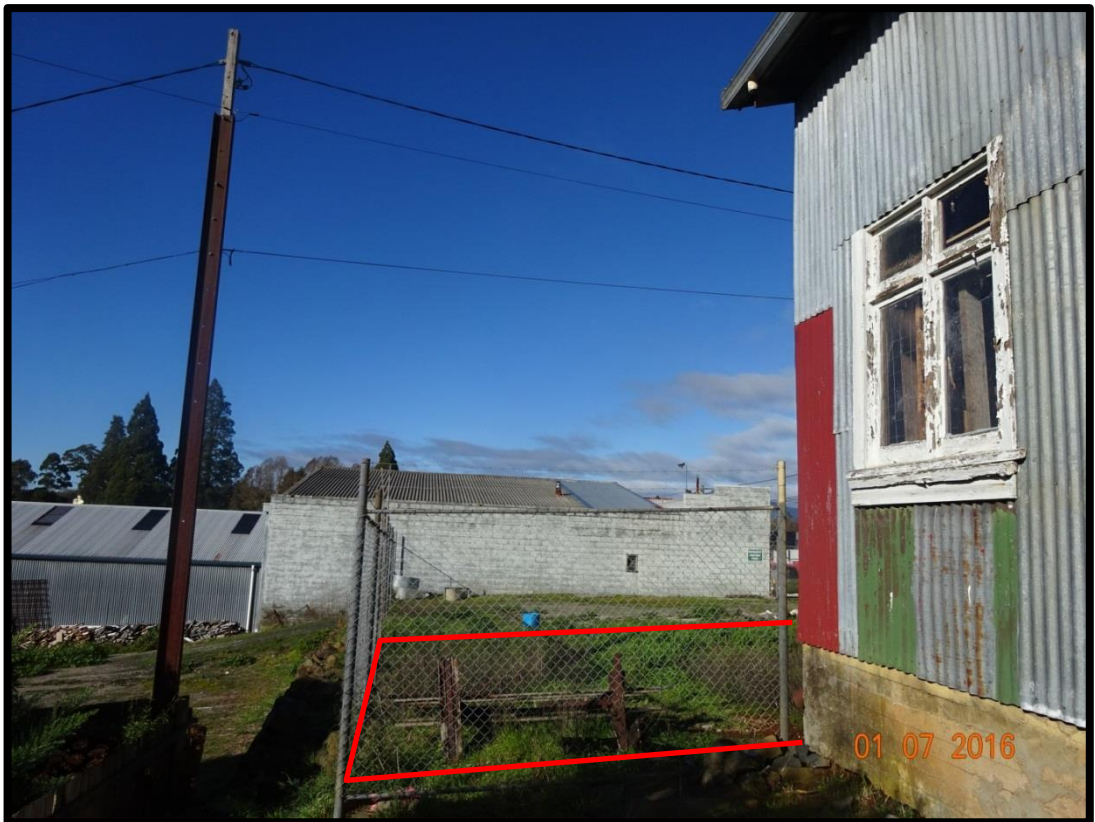
Photo 5: Location of proposed extension, looking south-east. Approx. footprint of extension in red.
