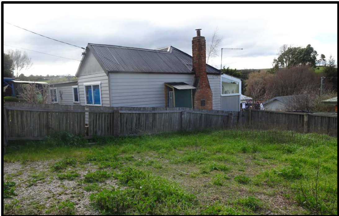
Photo 7: Adjoining residence at 13 West Barrack Street.
