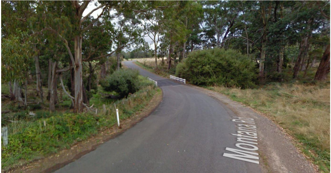
Image 2: Montana Road showing Bridge 164 looking south
