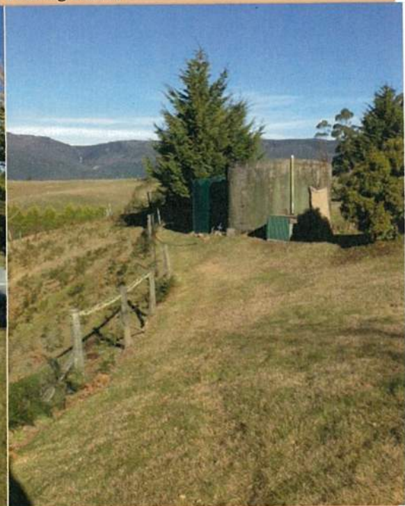
Existing water supply
