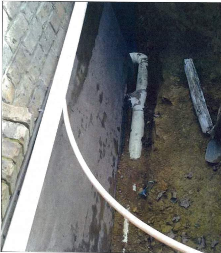
Figure 1 – Existing Plumbing at Cottage
