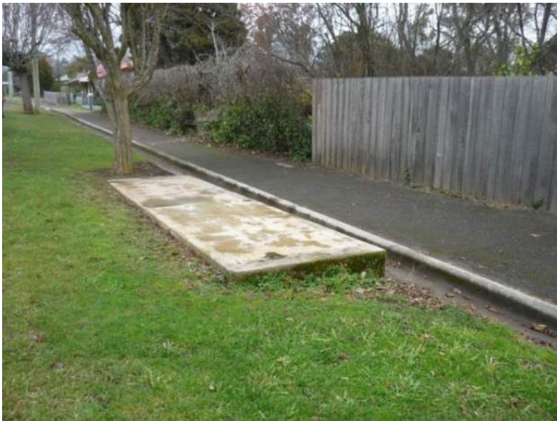
Photo 4: Existing concrete slab in William Street
