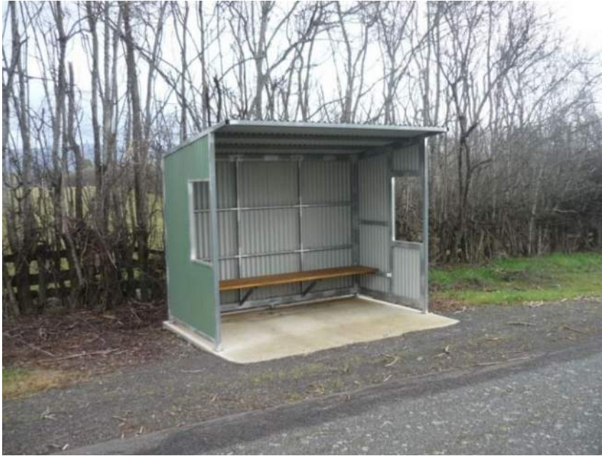
Photo 5: Existing shelter in Albuera Street
