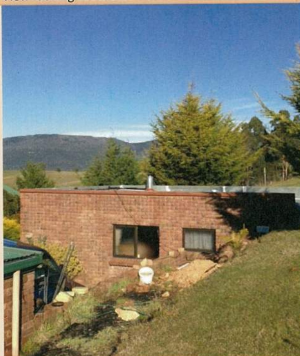
View looking south west from dwelling to accommodation building
