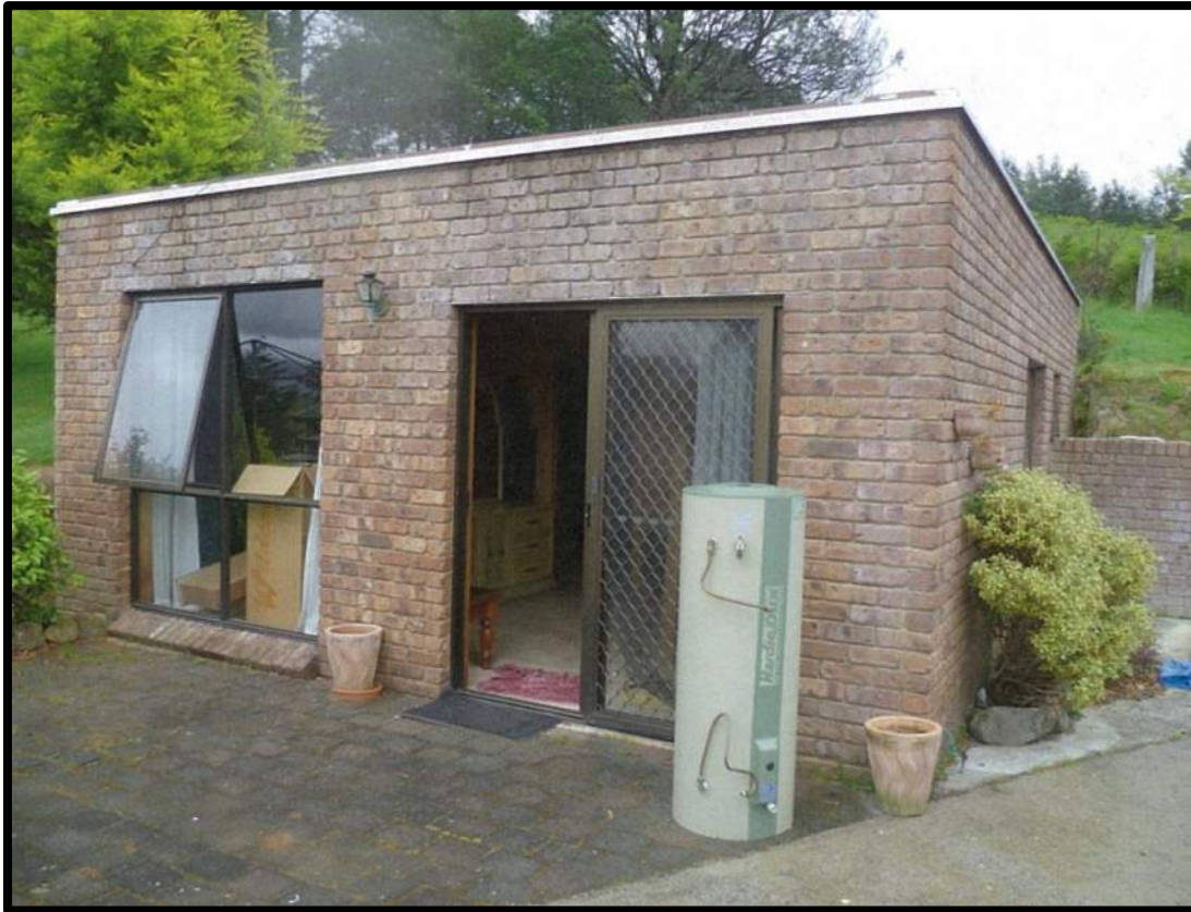
Photo 3: Outbuilding to be converted to visitor accommodation, viewed from internal driveway.
