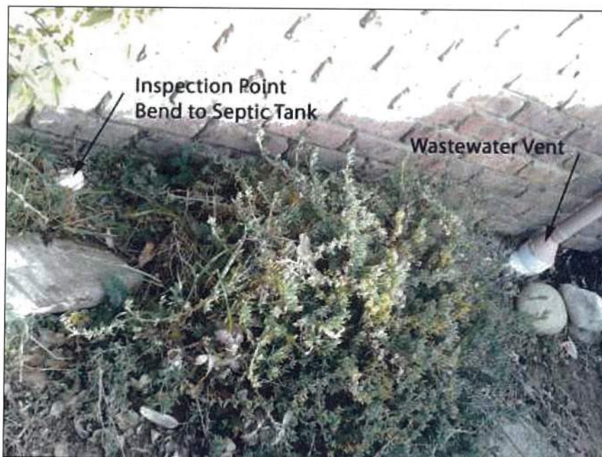
Figure 2 – Existing Plumbing at House
