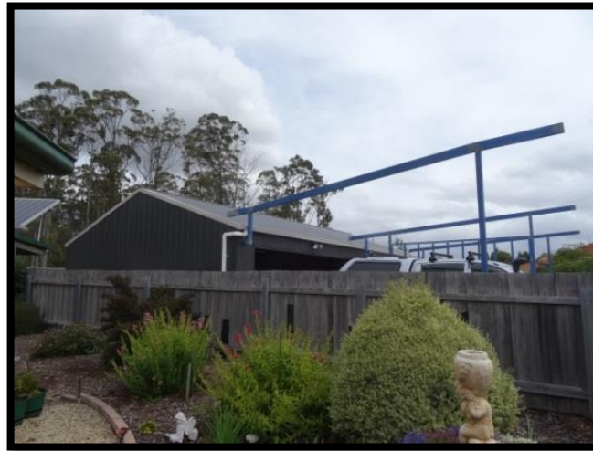
Photo 4: Photos from patio area of 4 Chelmsford Close.
