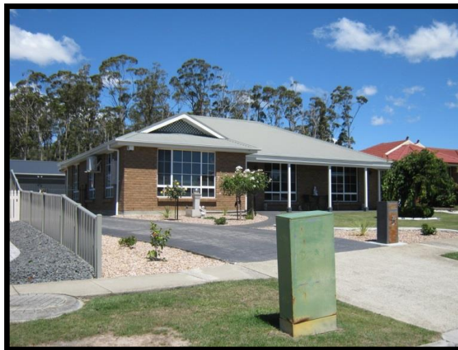
Photo 3: View of property from Cheltenham Way.
