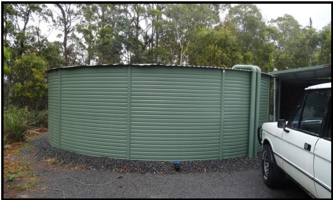
Photo 4: Proposed water tank.
