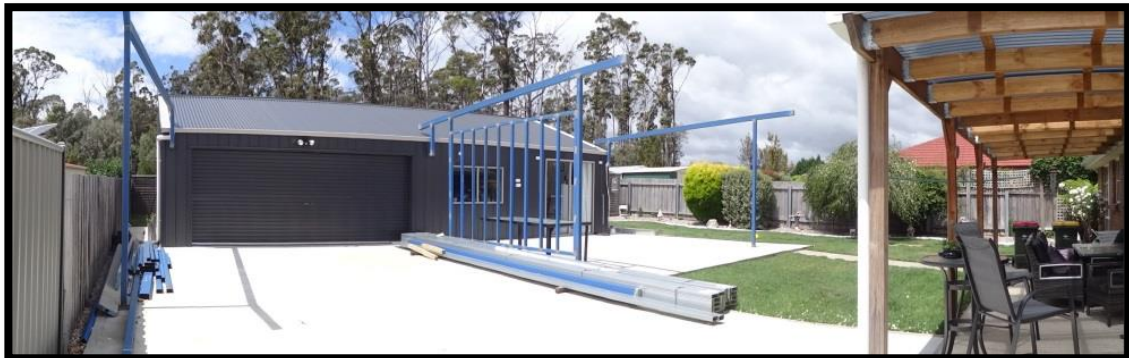
Photo 2: Outbuilding to be extended and commenced framework for the extension.
