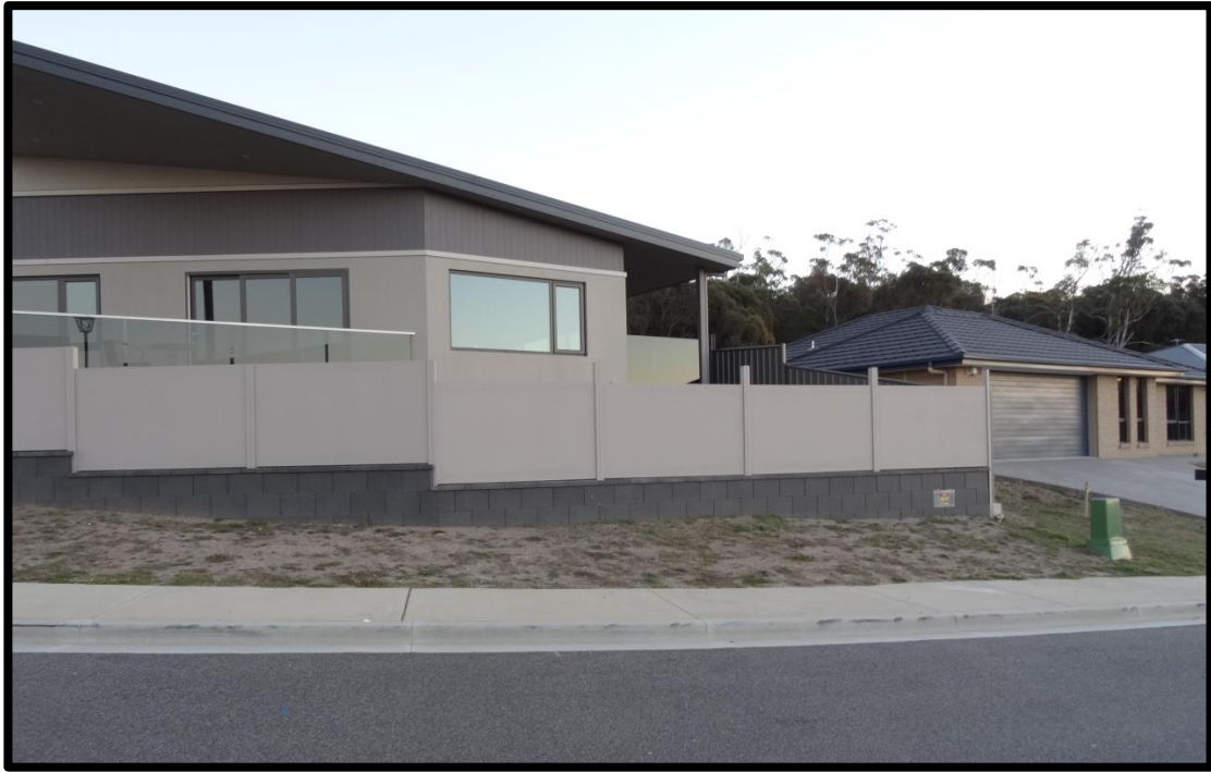
Photo 5: Existing 1.8m fence at 5 Classic Drive.
