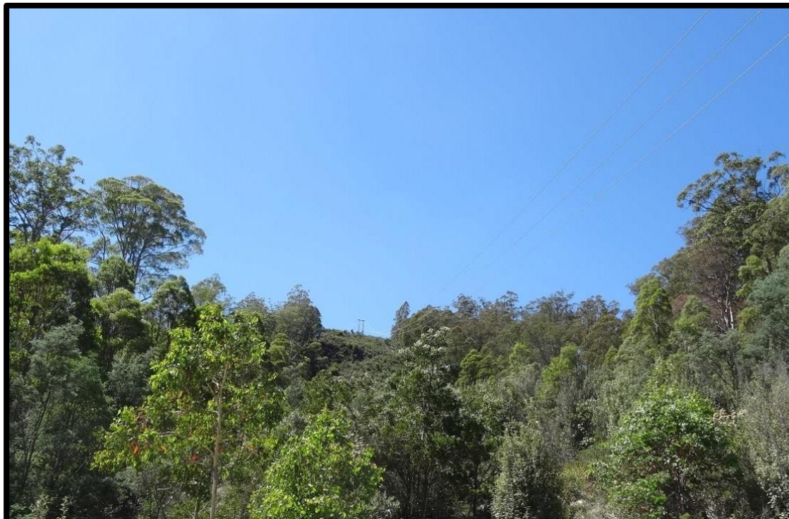
Photo 4: Existing transmission lines, adjacent to Rowallan Dam, looking north-east.
