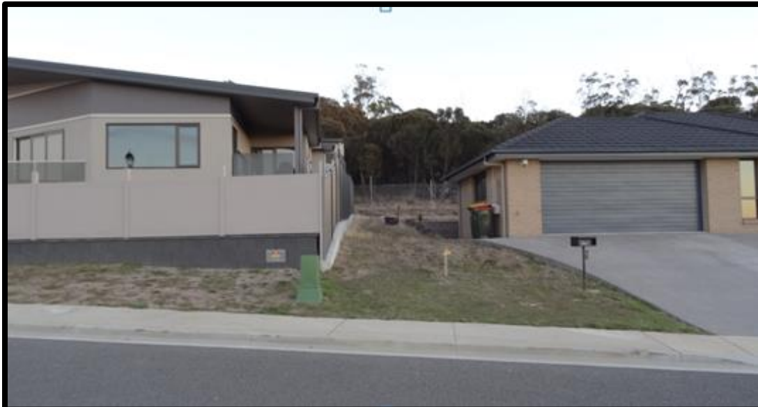
Photo 9: Existing visual bulk of 5 Classic Drive, compared to the existing dwelling at 7 Classic Drive.
