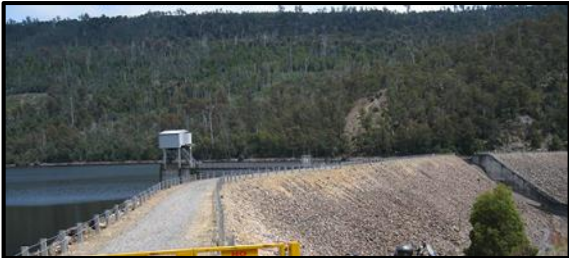
Photo 2: Rowallan Dam, looking west from Mersey Forest Road.
