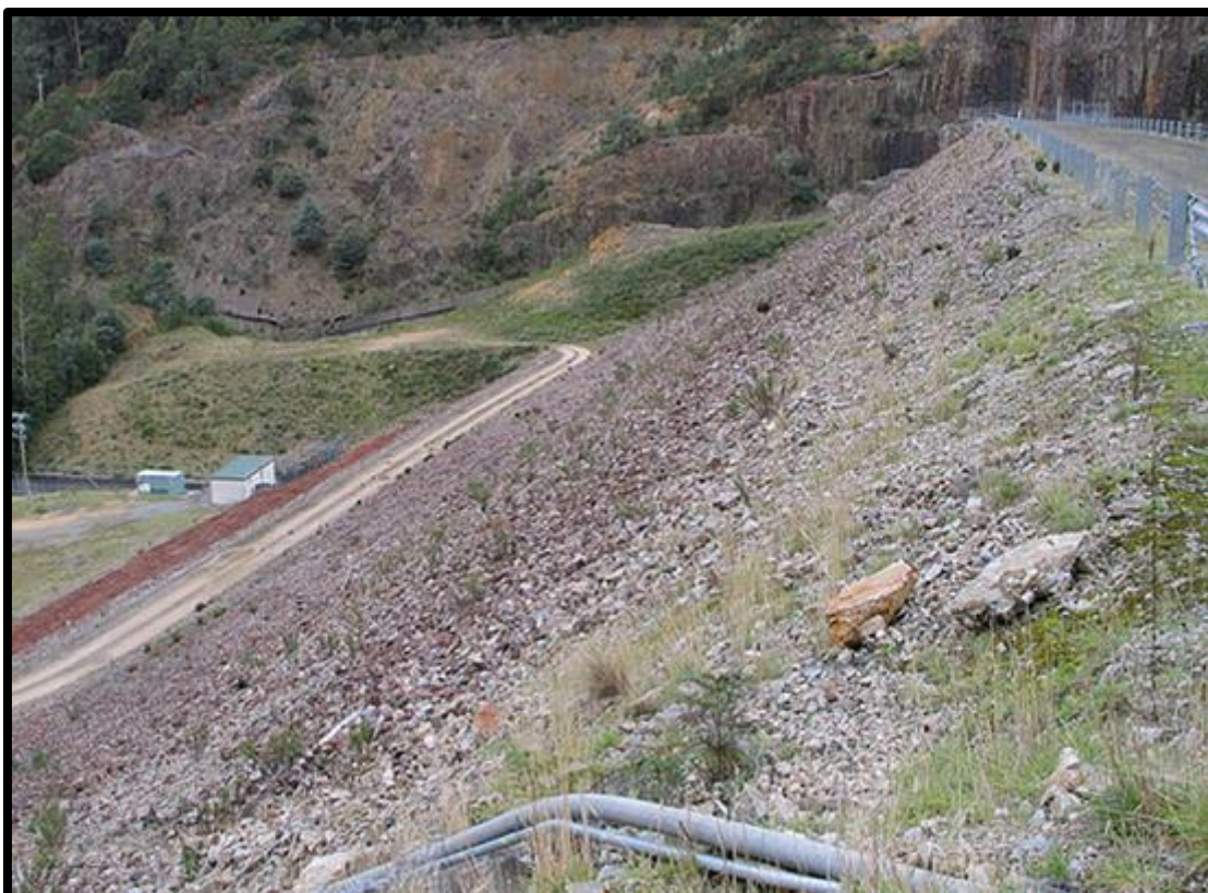
Photo 5: Parangana Dam and Power Station to the north-west of the development site, viewed from Mersey Forest Road.
