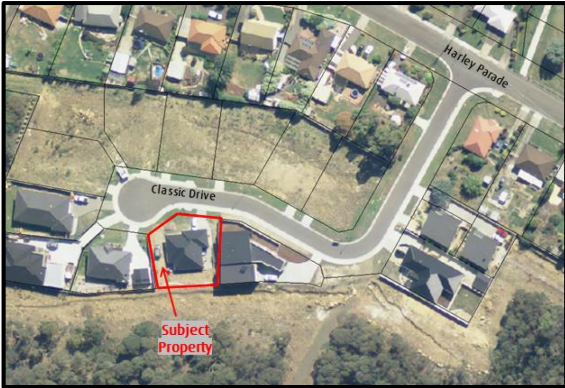
Photo 3: Aerial photo showing approximate location of the subject title.
