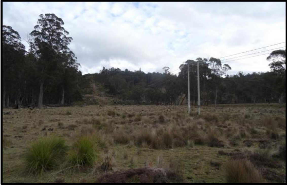
Photo 16: Existing transmission line corridor, looking south from existing shack at Dublin Plains
