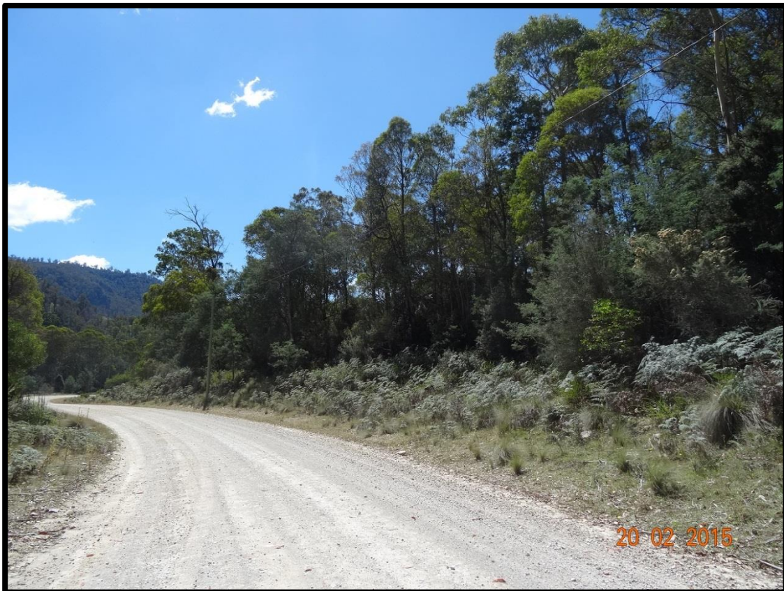
Photo 13: Mersey Forest Road to the north of Lake Rowallan, showing existing transmission lines.
