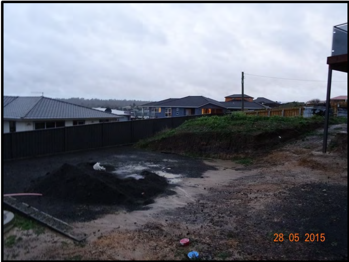
Photo 3: Site of development, looking south-west within the subject lot, showing fill to be retained and building platform.
