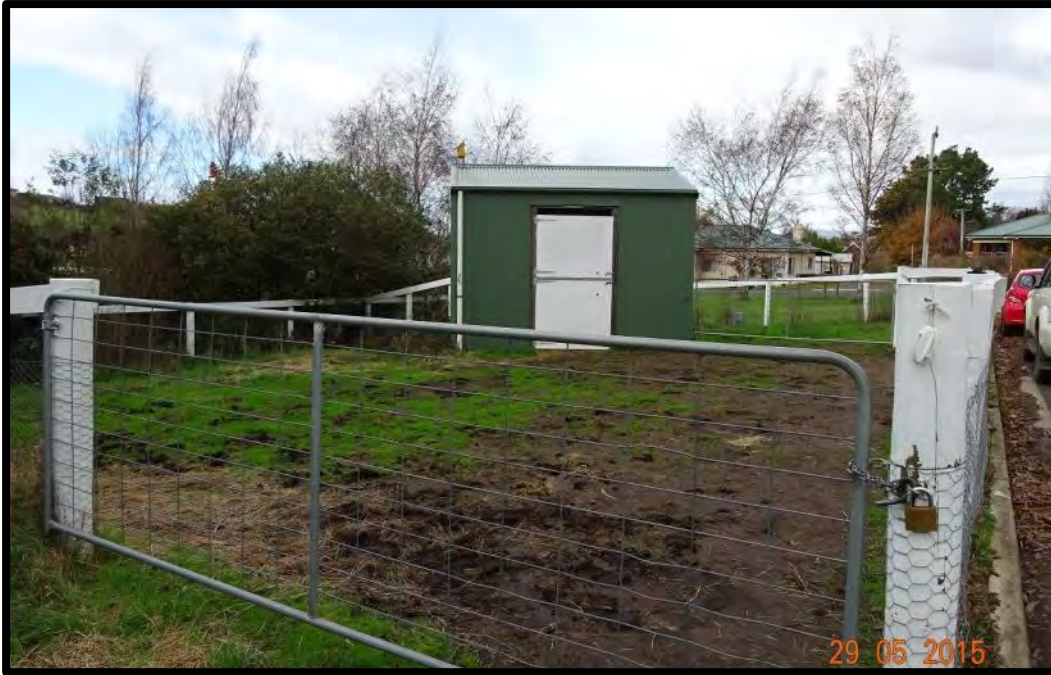
Photo 4: Building 4, stable constructed without a permit.
