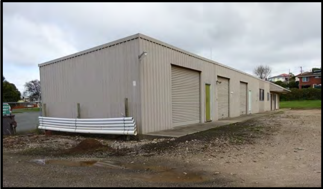
Photo 2: Building 2 to be used as horse surgery, recovery, administration and amenities.
