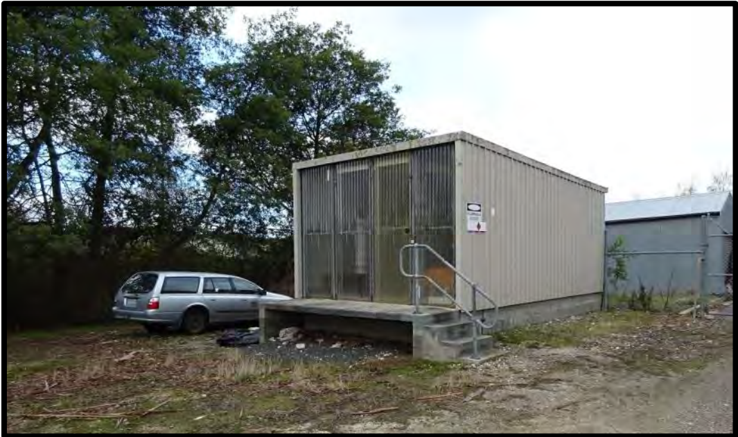
Photo 3: Building 3, bulk store.
