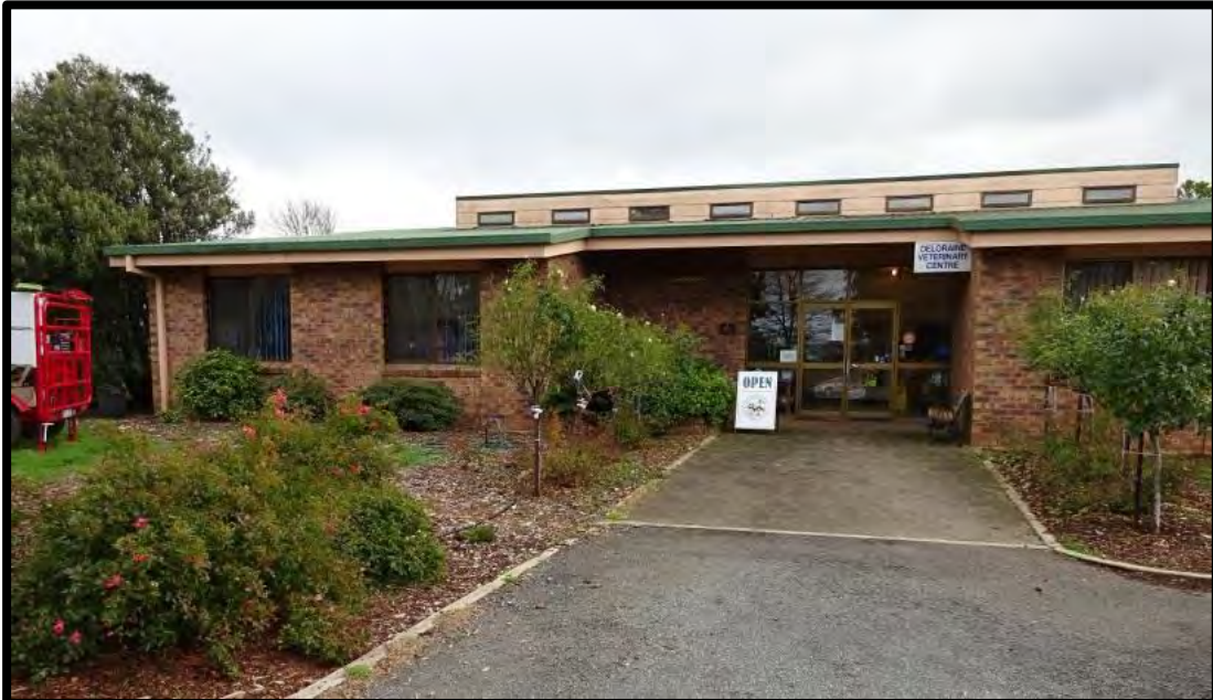
Photo 7: Building 6, the existing clinic.
