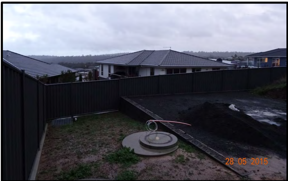
Photo 4: Site of development, looking south within the subject lot, showing existing retaining wall and building platform.
