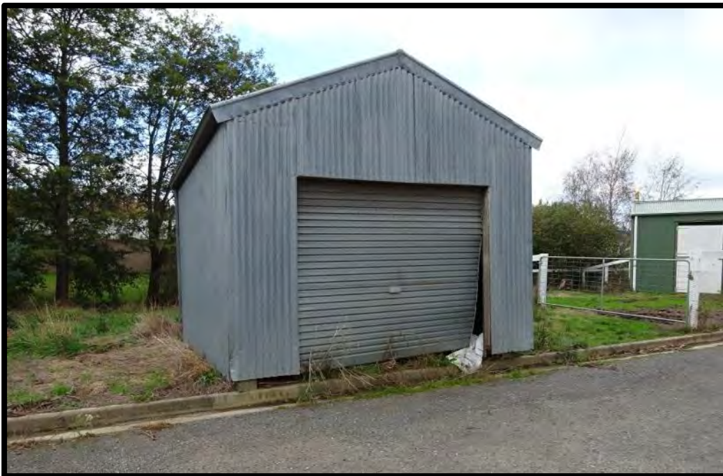
Photo 5: Building 5, constructed without a permit, to be used as a store and relocated.
