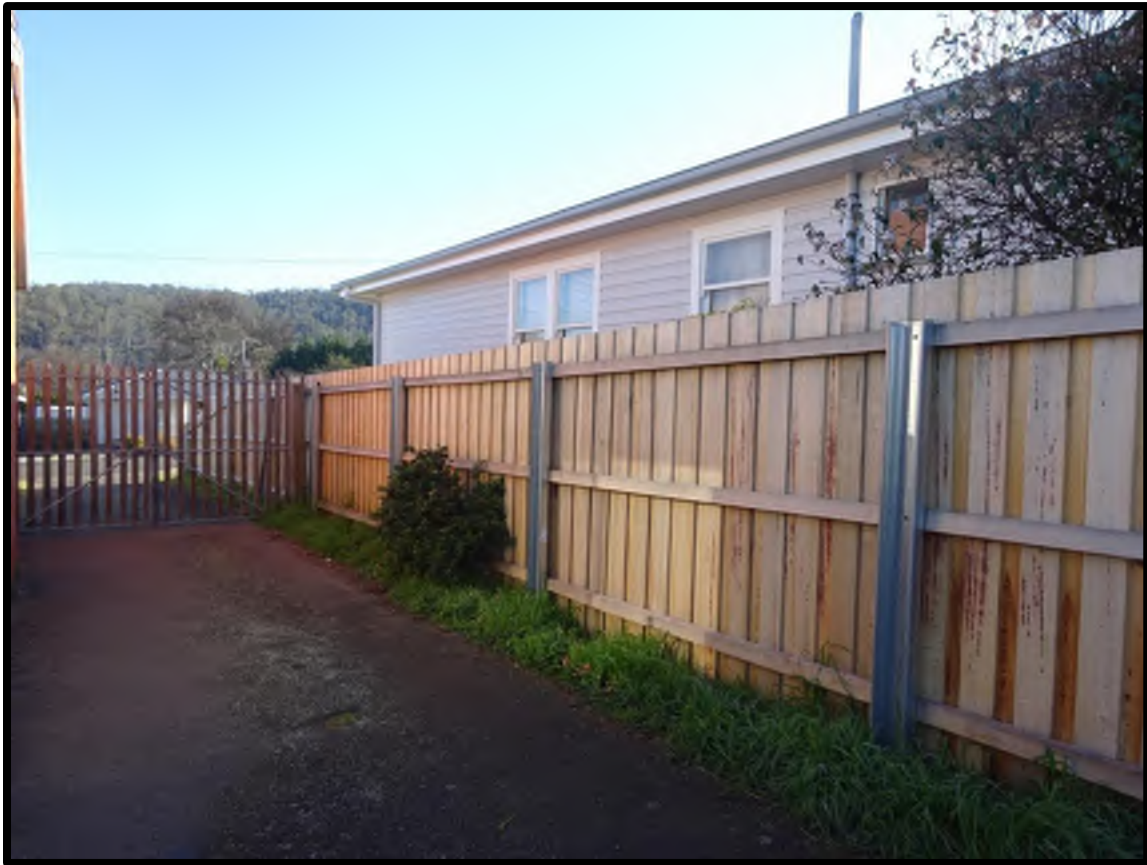
Photo 6: showing the side boundary fence with 3 Reibey Street.
