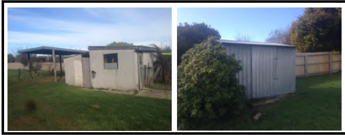
Photos 4 & 5: buildings to be demolished.
