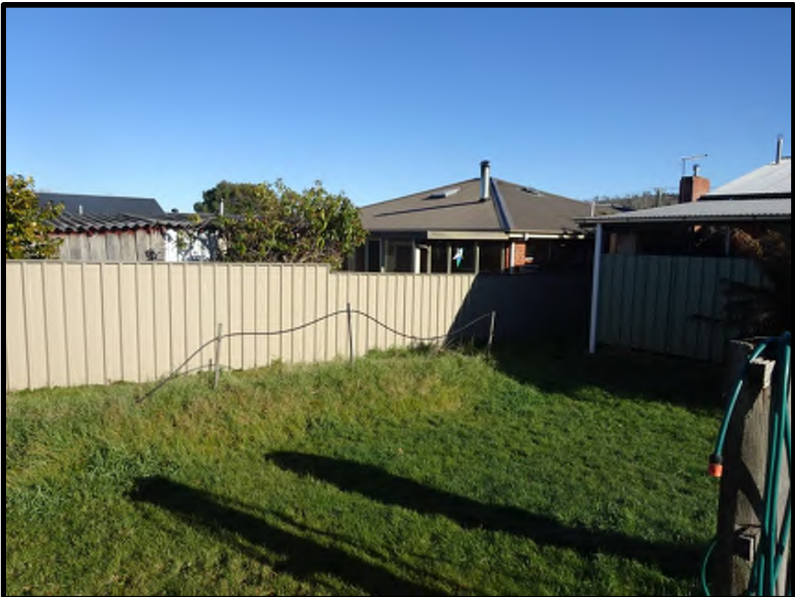
Photo 7: showing the side boundary fence with 7 Reibey Street.
