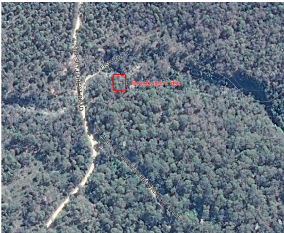
IMAGE 2: Aerial image of power generation site and environs.
