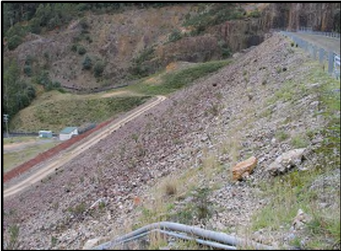
Photo 5: Parangana Dam and Power Station to the north-west of the development site, viewed from Mersey Forest Road.
