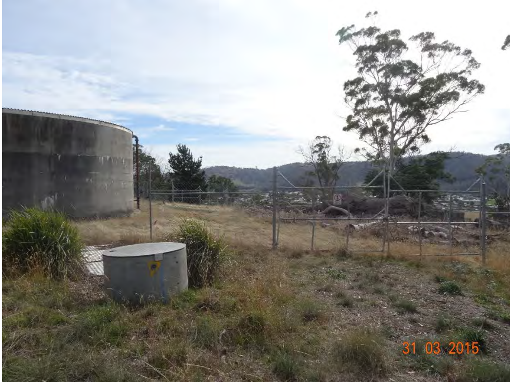
Photograph 17: TasWater Reservoir, looking west over Hadspen.
