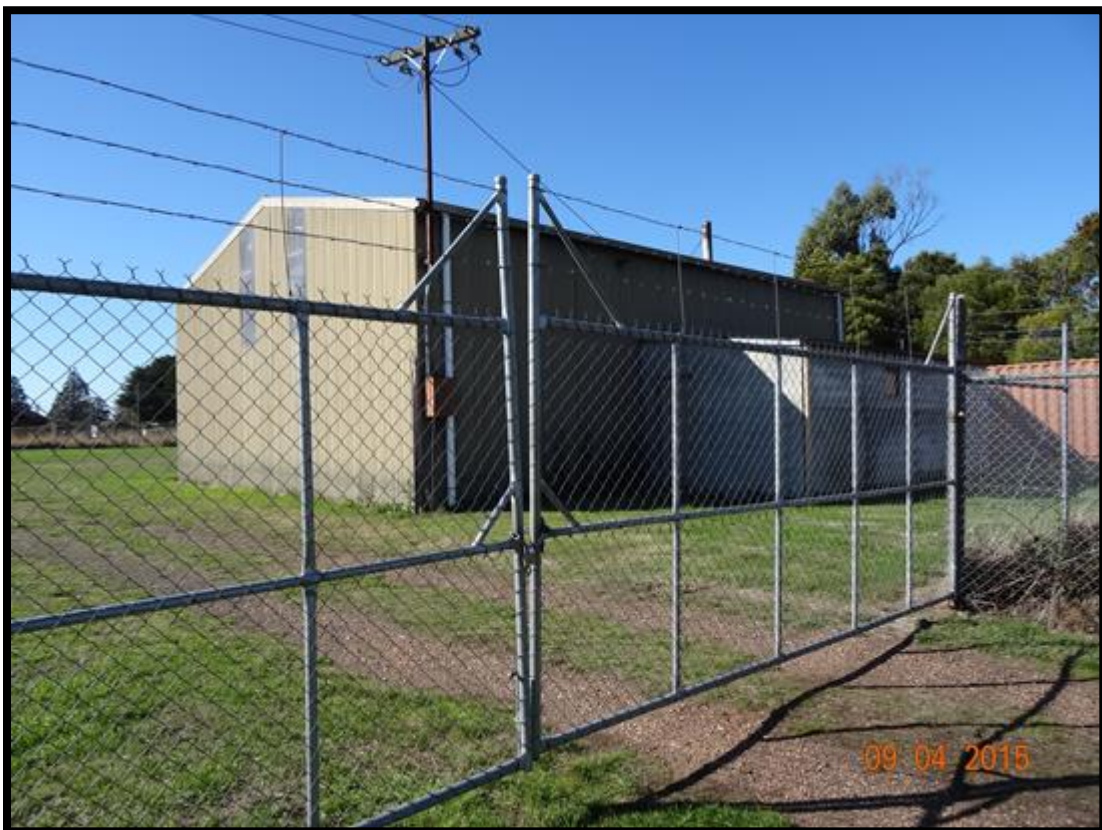
Photo 3: showing building (Shed B) to be retained
