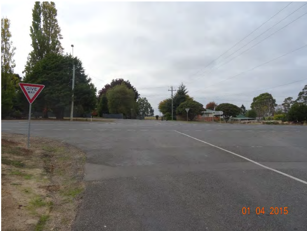
Photograph 11: Scott Street junction with Meander Valley Road, showing access into the site beyond
