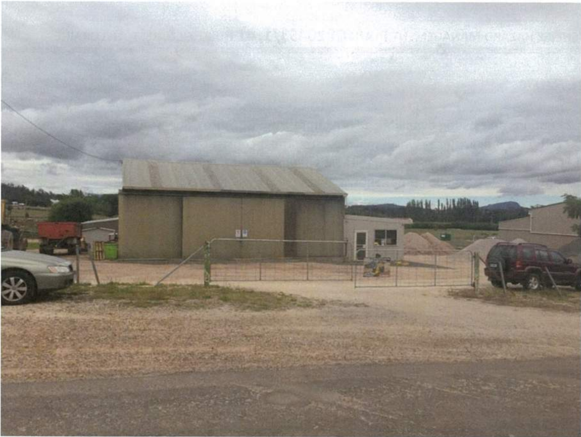
Plate 7: Light Industrial zoned land to the south west of Lot 2.
