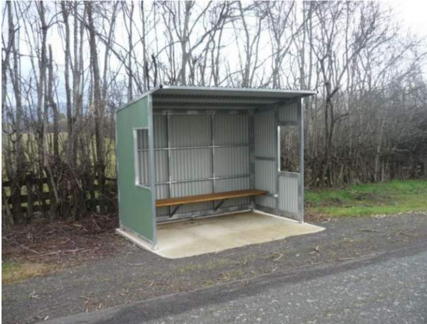
Photo 5: Existing shelter in Albuera Street
