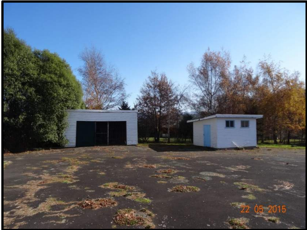
Photo 2: Ancillary buildings (storage shed and toilet block) to be demolished, looking west from within the title.
