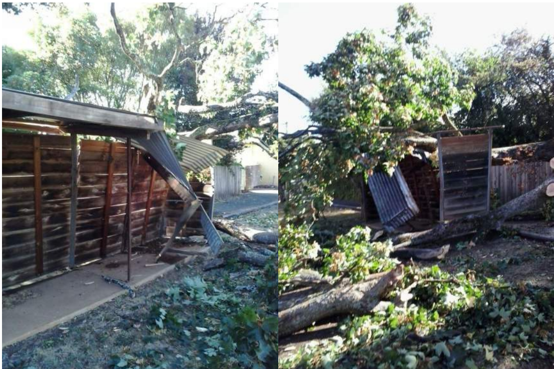
Photo 1 and 2 : Damage to existing timber bus shelter
